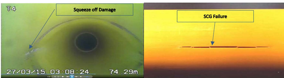
Figure 4.9: Internal Squeeze-off Damage (Left) and SCG Failure (Right)
