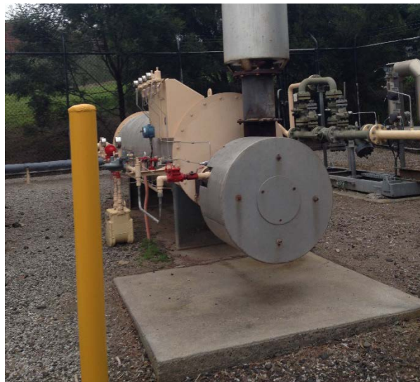
Figure 2: WBH Slab Edge Exposed – Trip Hazard
