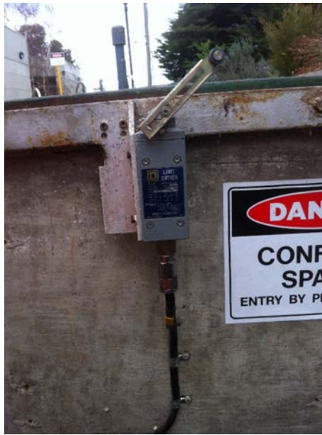
Figure B.3 – Non-certified electrical equipment – non-compliant
