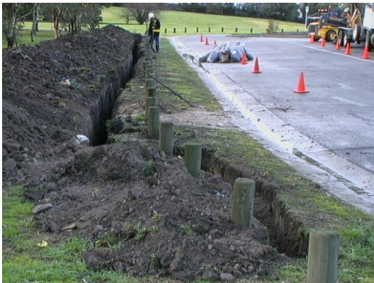
Figure 1.2: Installation of an Anode Bed
