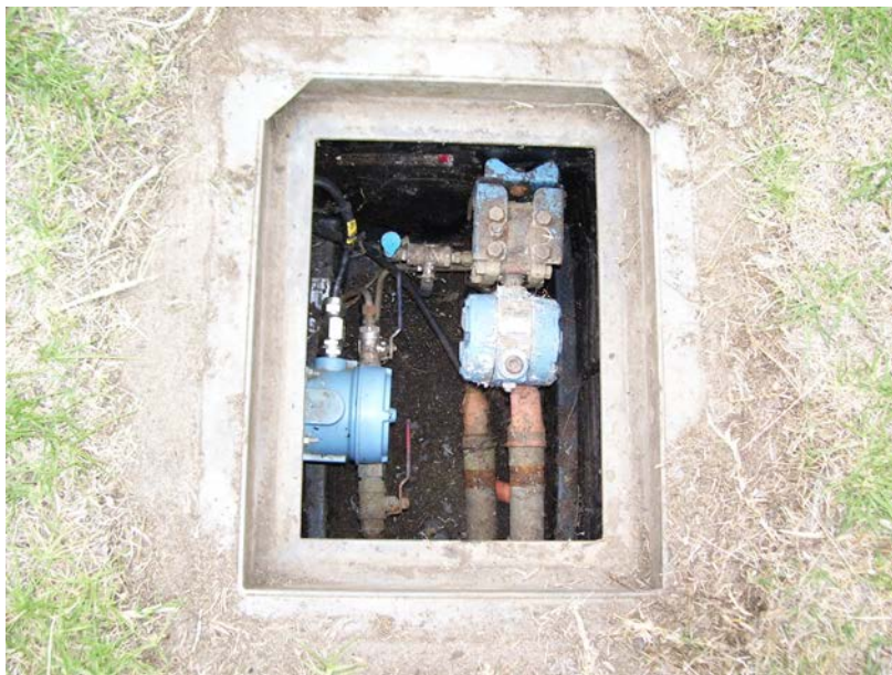
Figure B.2 – Corroded equipment unable to be opened
