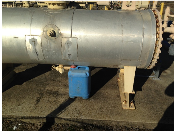
Figure 1.1: No Earthing on Heater, Rosedale City Gate
