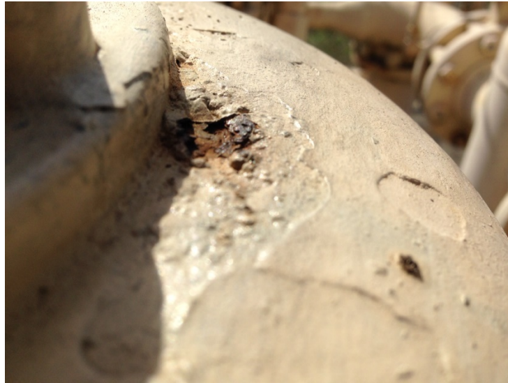
Figure 1.2: Delaminating Paint & Corrosion on I&C Meter Set Pipework
