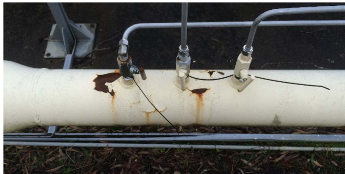
Figure 1.2: Delaminating Paint & Corrosion on I&C Meter Set Pipework
