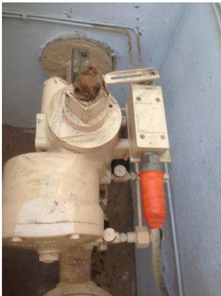
Figure B.1 – Painted switch – non-compliant
