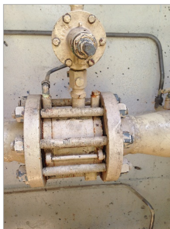
Figure 1.1: Typical Installed Grove 82 Regulator Unit
