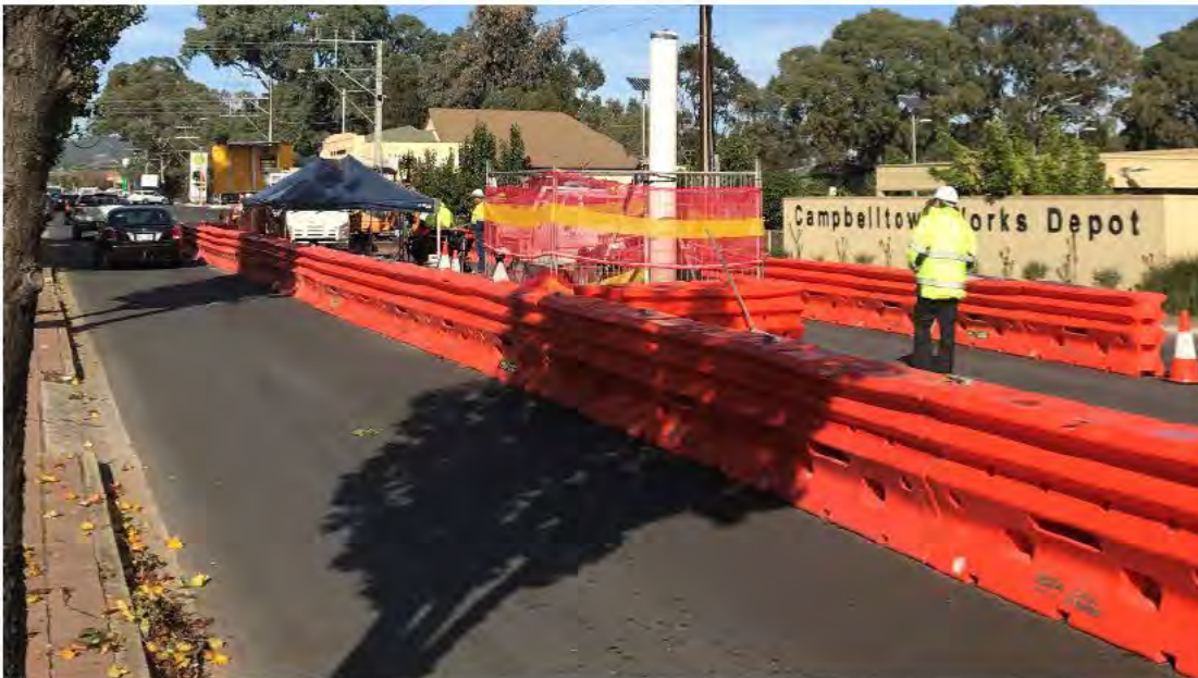
Figure 1.1: Isolation and replacement of TP valve 1034, March 2018
