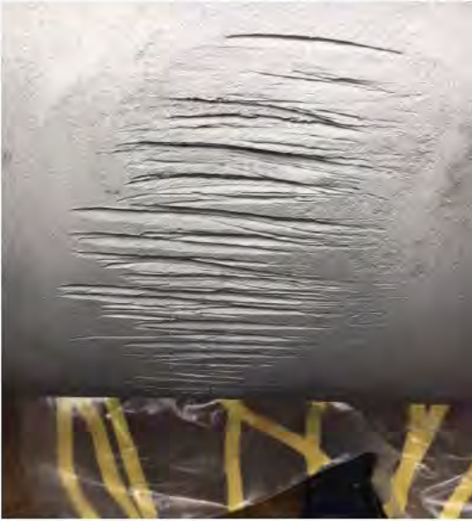
Figure 1.3: Damage on [REDACTED] detected by DCVG survey and excavation
