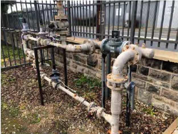
Figure 1.3: I&C meter set corrosion – soil/air interface
