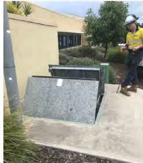
Figure 1.3: Example of proposed steel butterfly lid
