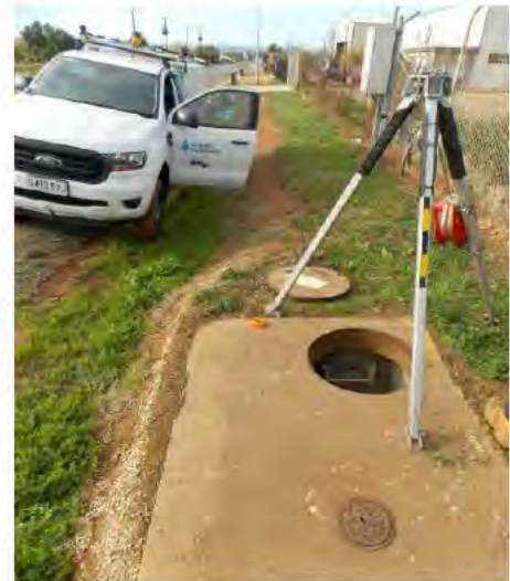
Figure 1.1: Example of a Gatic concrete DRS lid
