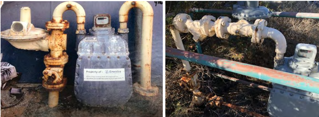
Figure 1.1: I&C meter set – corrosion of valve and regulator
