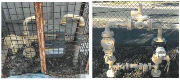
The bypass line for our 686 customers with I&C rotary/turbine meter sets typically includes one or two isolation valves that separate the upstream high (350 kPa) or medium (90 kPa) pressure from the downstream customer supply pressure. During maintenance of the duty stream, these bypass line isolation valves can be opened and manually throttled and monitored to maintain gas supply to the customer, while the duty stream on the meter set is shut down.
