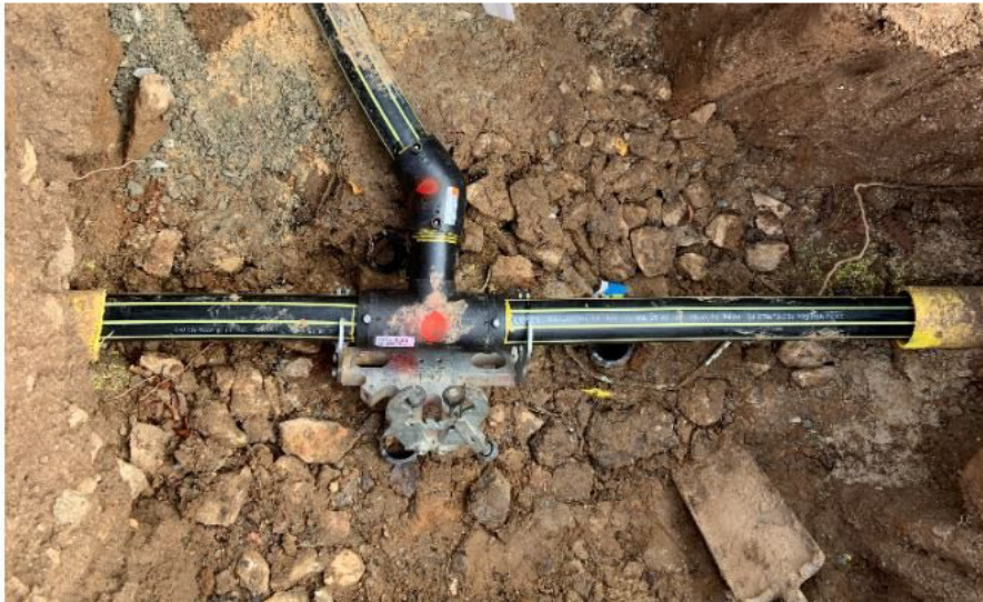
Figure 1: Inserted main with service connection
