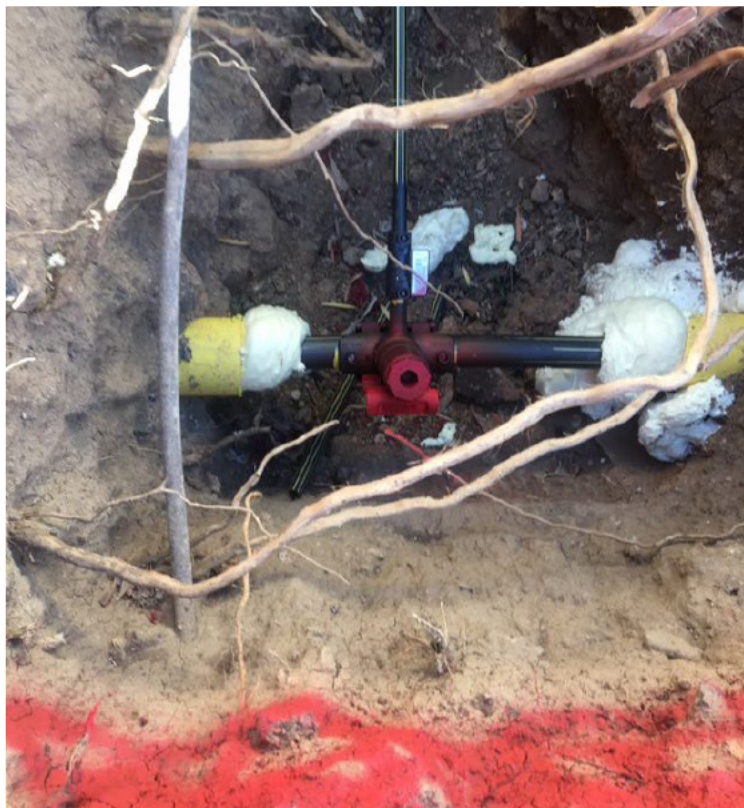
Figure 2: Inserted main with existing HDPE main removed
