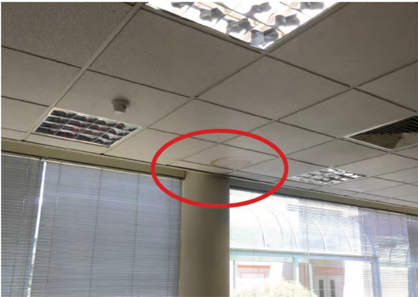
Photo 19. Water damage to office
