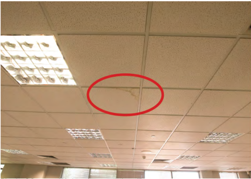
Photo 12. Water damage to office
