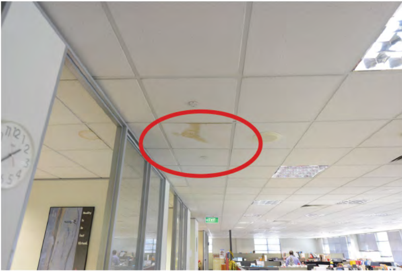
Photo 9. Water damage to office
