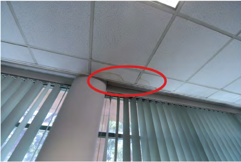
Photo 24. Water damage to lunch room
