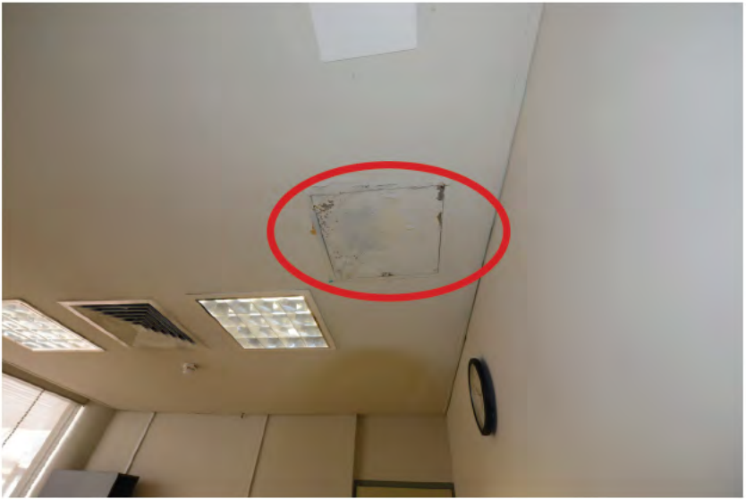
Photo 21. Water damage to first aid room
