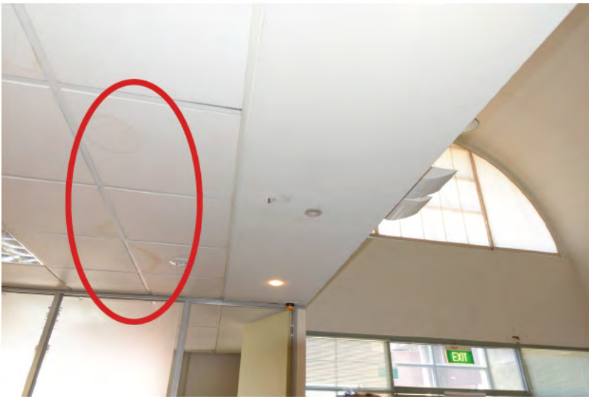
Photo 4. Water damage to reception
