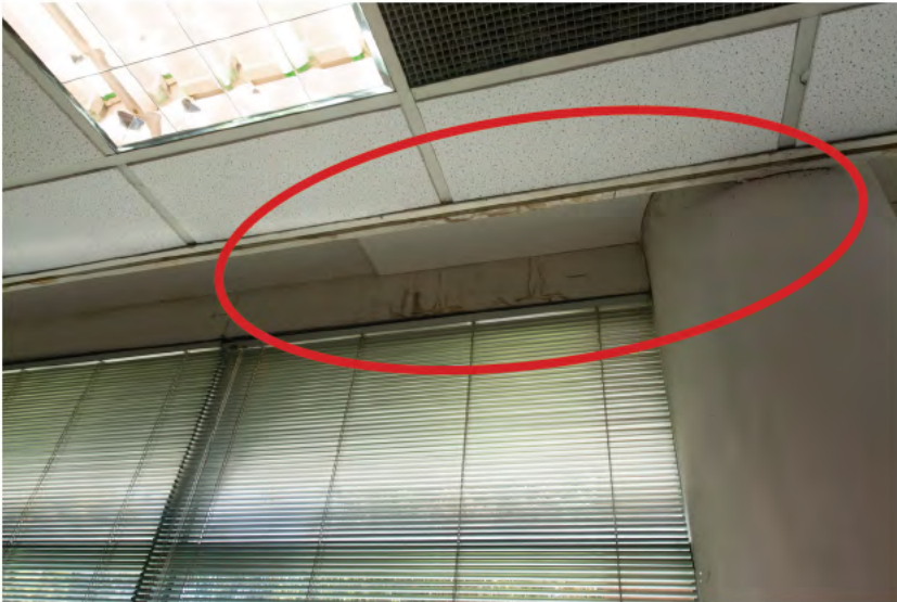
Photo 7. Water damage to office
