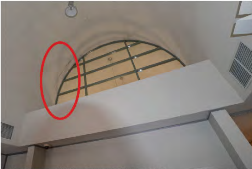
Photo 1. Water damage to reception
