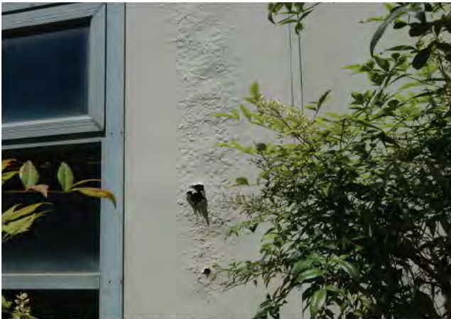
Photo 40. Insulated panels rusting
