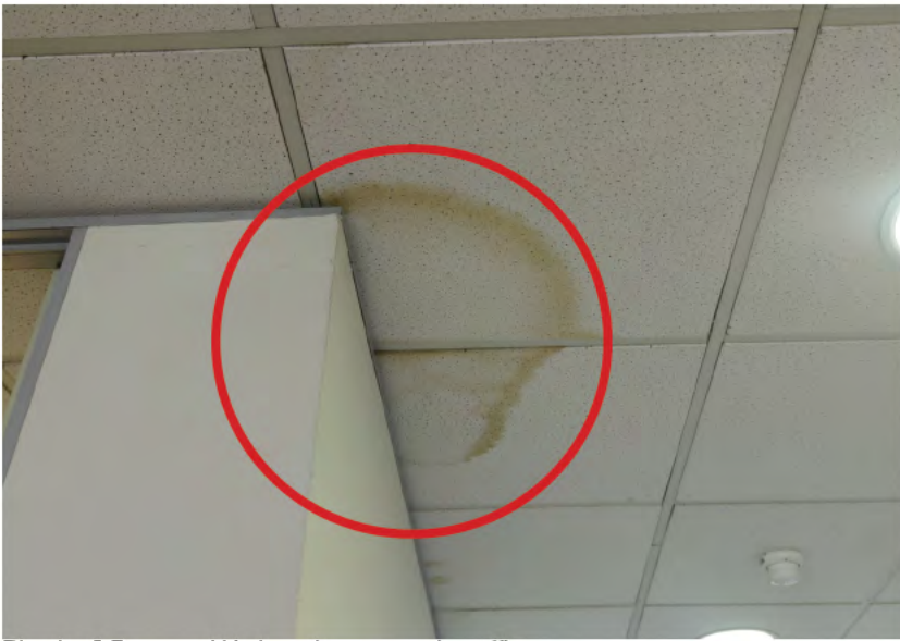
Photo 15. Water damage to office
