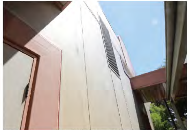
Photo 41. Insulated panels rusting
