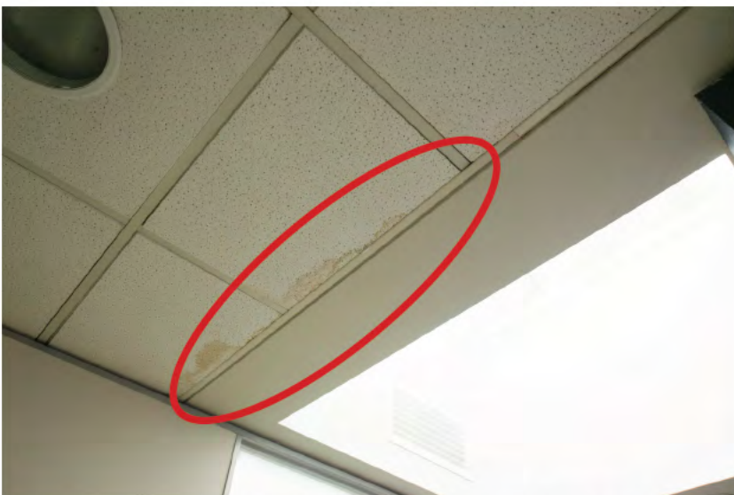
Photo 20. Water damage to meeting room corridor
