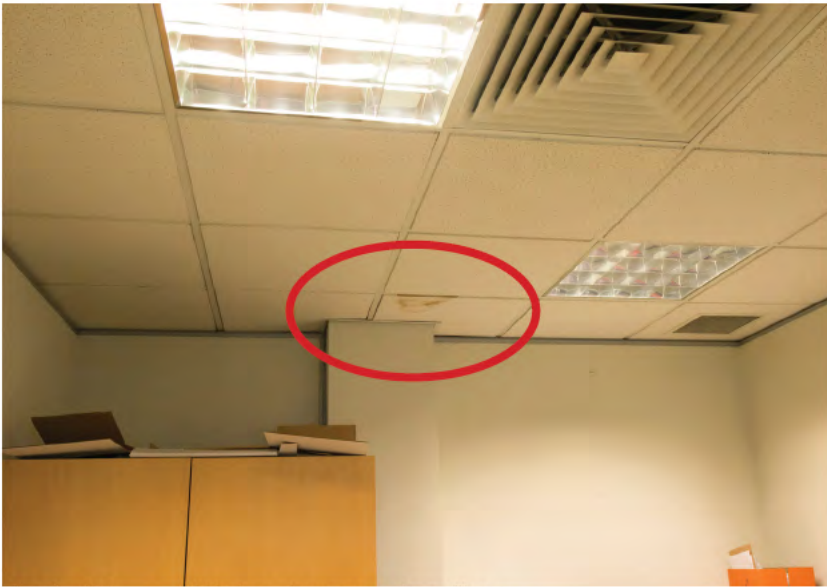
Photo 10. Water damage to office
