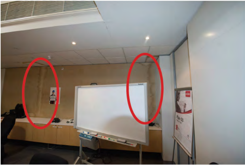
Photo 3. Water damage to boardroom
