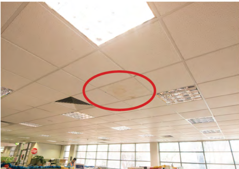
Photo 11. Water damage to office
