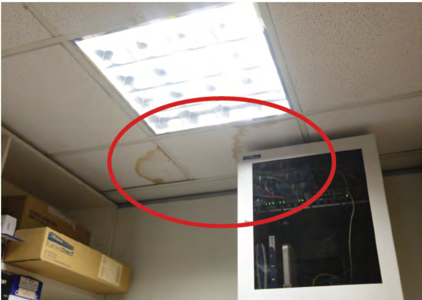
Photo 18. Water damage to comms area
