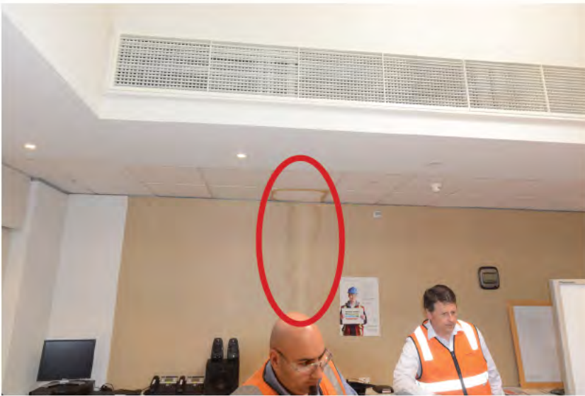
Photo 2. Water damage to boardroom
