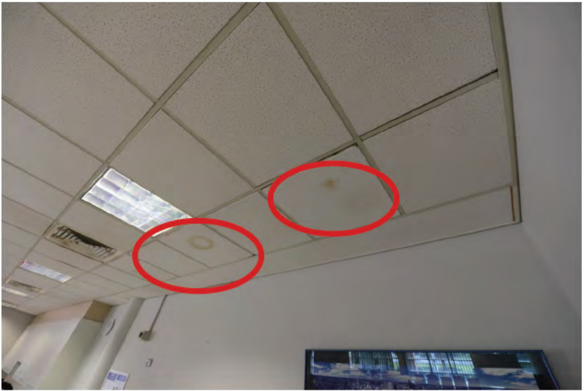
Photo 22. Water damage to lunch room
