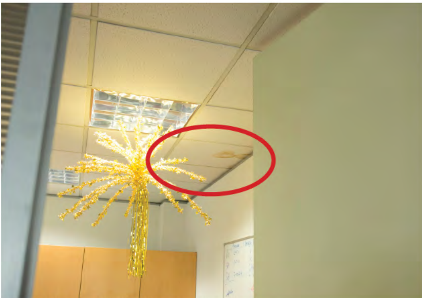
Photo 14. Water damage to office
