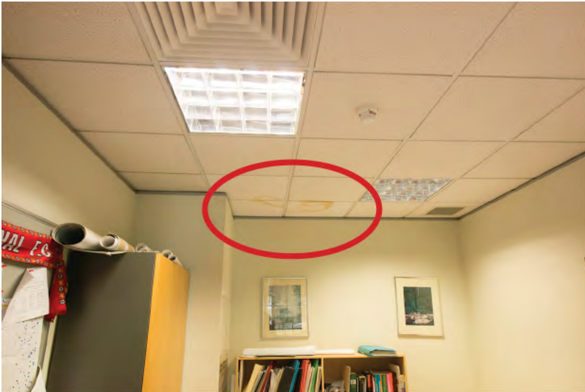
Photo 8. Water damage to office
