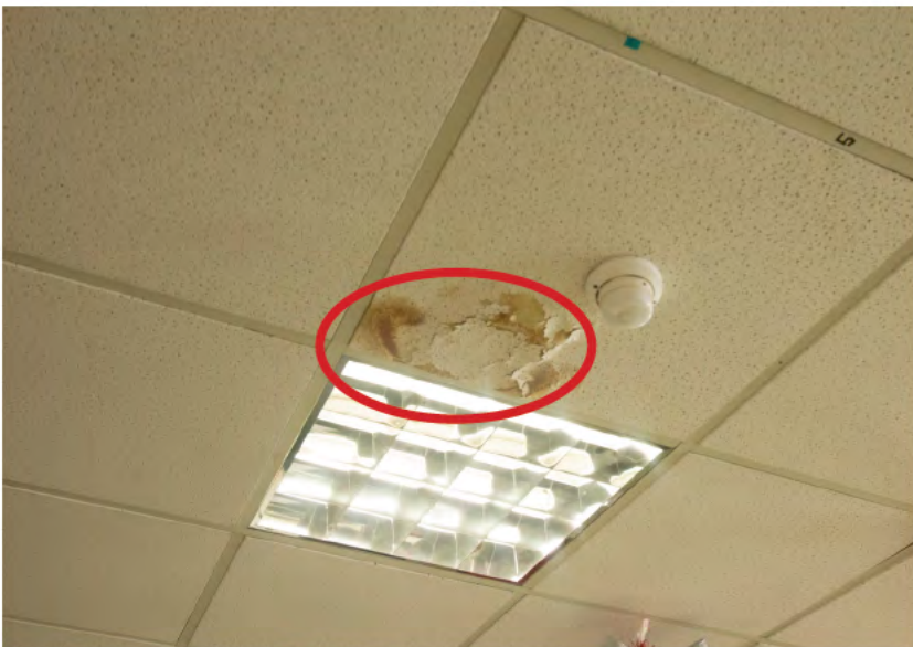
Photo 13. Water damage to office
