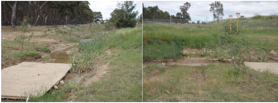
Fig 2 Undermined scouring protection slab Melbourne Water Course National Drive
