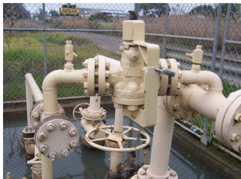
Fig 3: Graydens Road line valve installation
