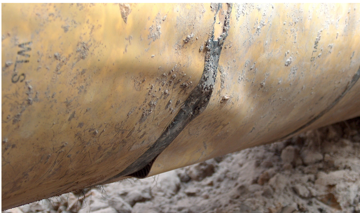
Image 2: The disbonded heat shrink sleeve is clearly evident on visual inspection
