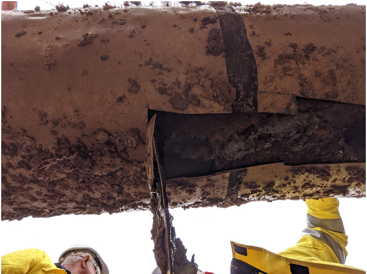
Image 4: Pipe condition under disbonded coating
