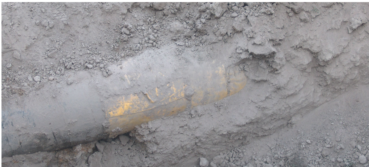
Image 1: Transition from original coal tar to the yellow heat shrink sleeve applied by the G&F Corporation.
