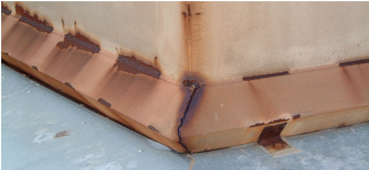
Figure 1 - Exhaust stack cracking
