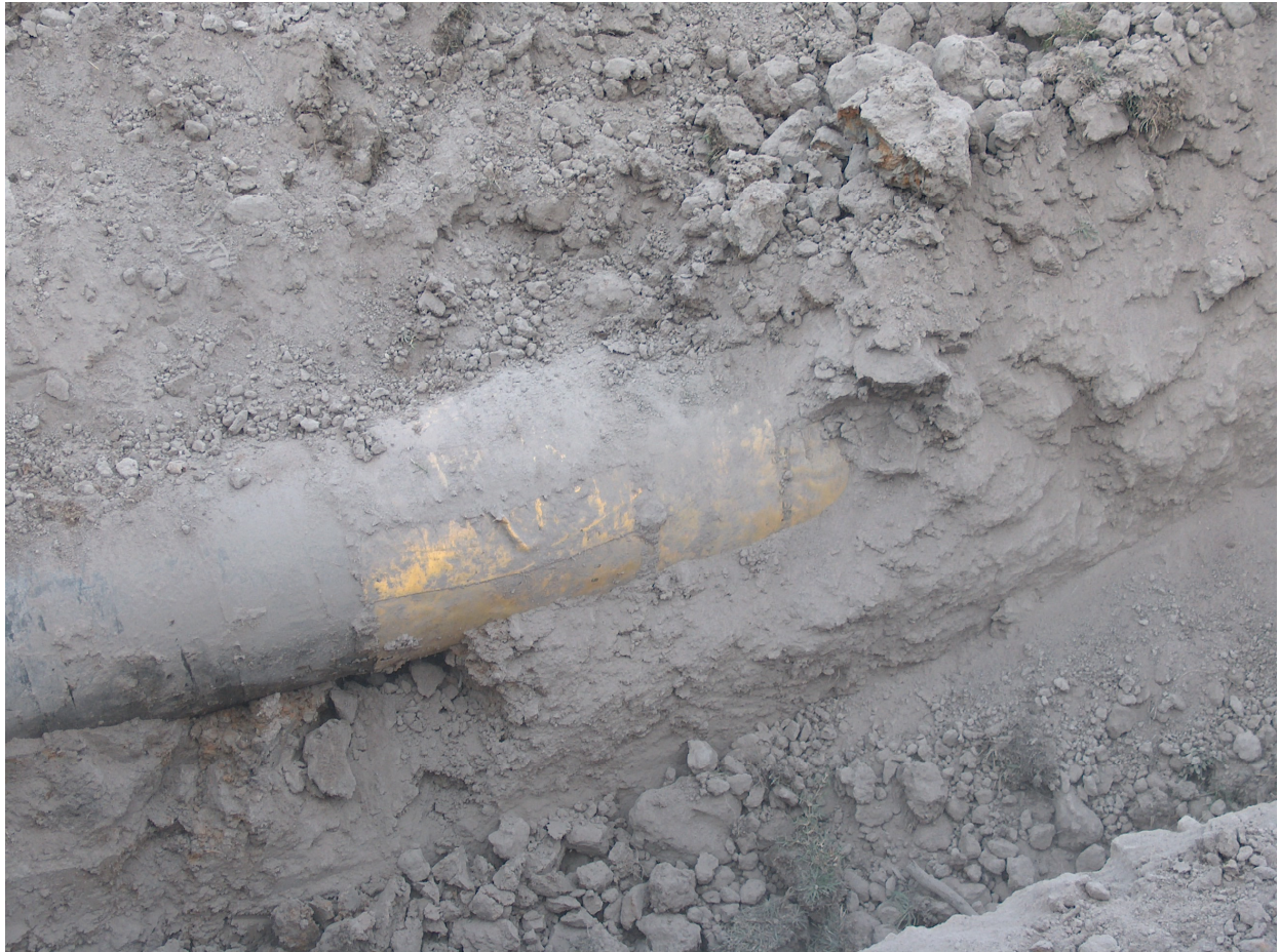
Image 1: Transition from original coal tar to the yellow heat shrink sleeve applied by the G&F Corporation.
