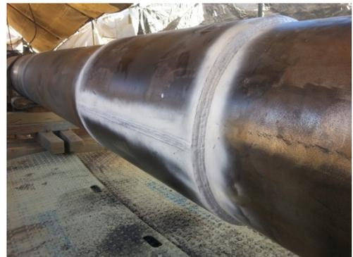
Engineering assessment recommended installing a Type B fully welded split sleeve to encase the crack for pressure retainment. This repair sleeve provides strength to fully support the pipeline and reinforce the longitudinal stresses in the axial direction along the pipeline required for a crack found in the circumferential direction.
