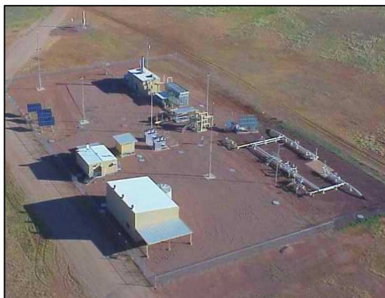
Morney Tank Compressor Station
