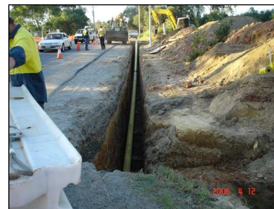
APT Allgas Network – steel main construction
