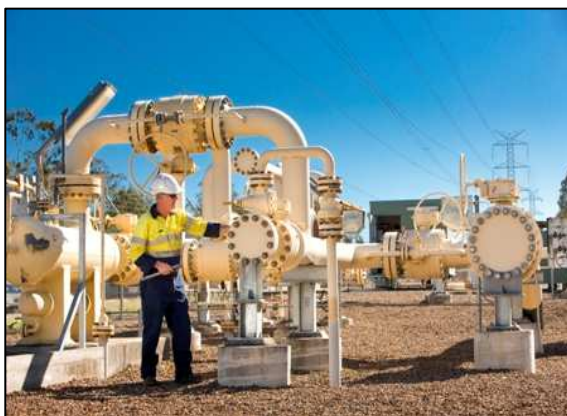
Ellengrove Gate Station – gas from Roma Brisbane Pipeline enters APT Allgas Network
