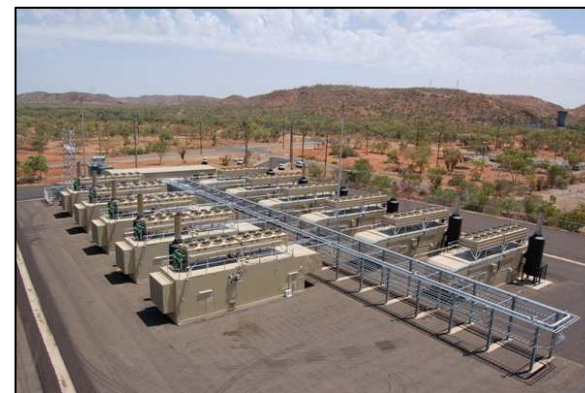
X41 Power Station, Mt Isa - EII
