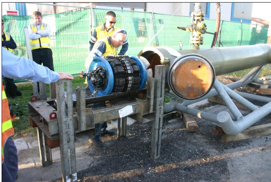
Figure 1: Example of Intelligent Pig in Launcher
