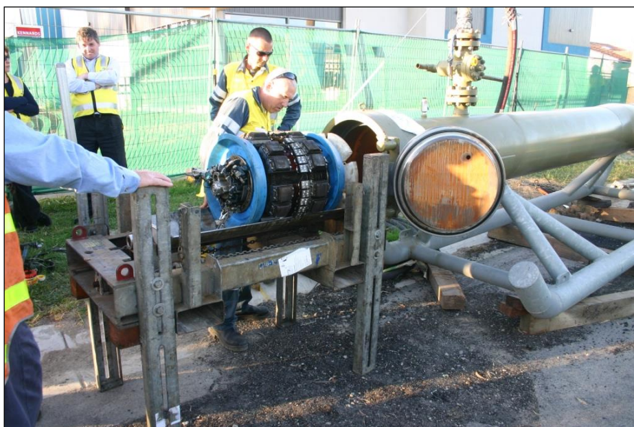
Figure 1: Example of Intelligent Pig in Launcher
