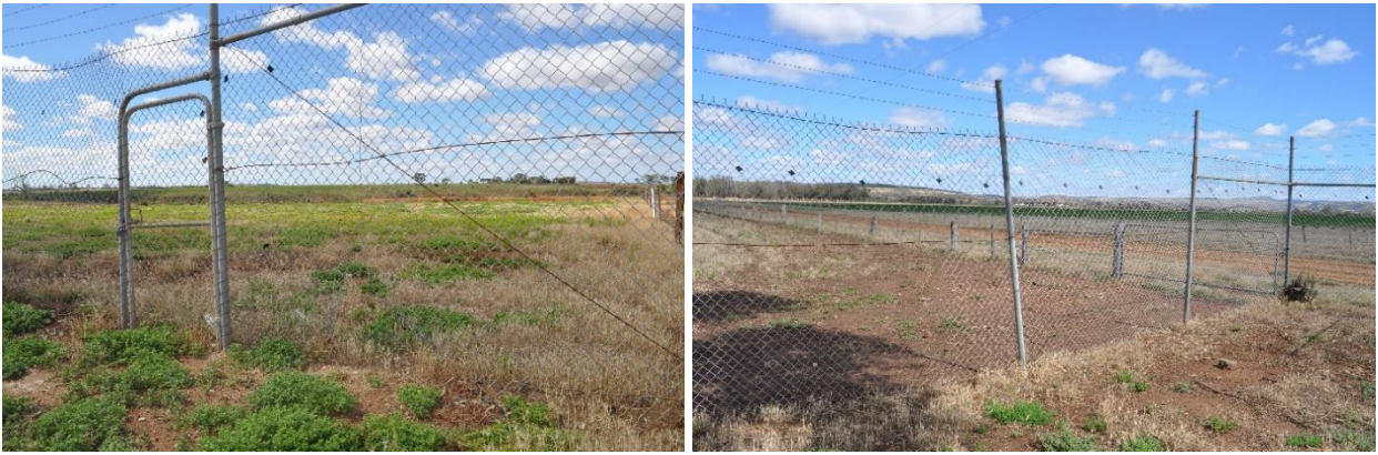
Figure 20 – Chain wire mesh fence
