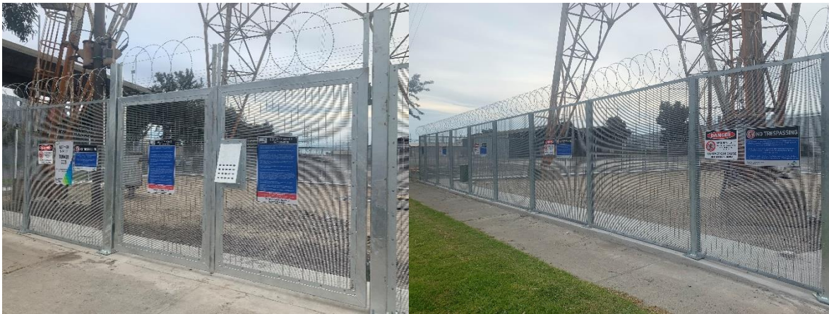
Figure 21 – High security fencing
