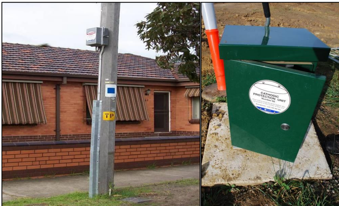
Figure 5: Typical CPU Installation
