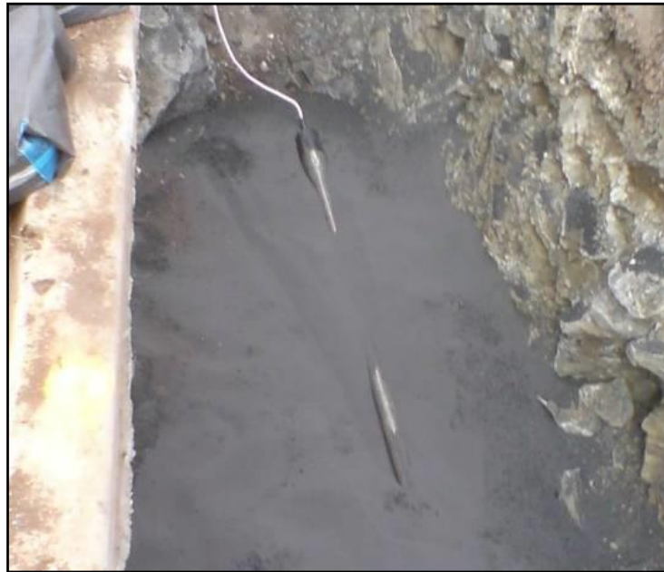
Figure 6: A Small Anode Bed Installation (Single Anode)
