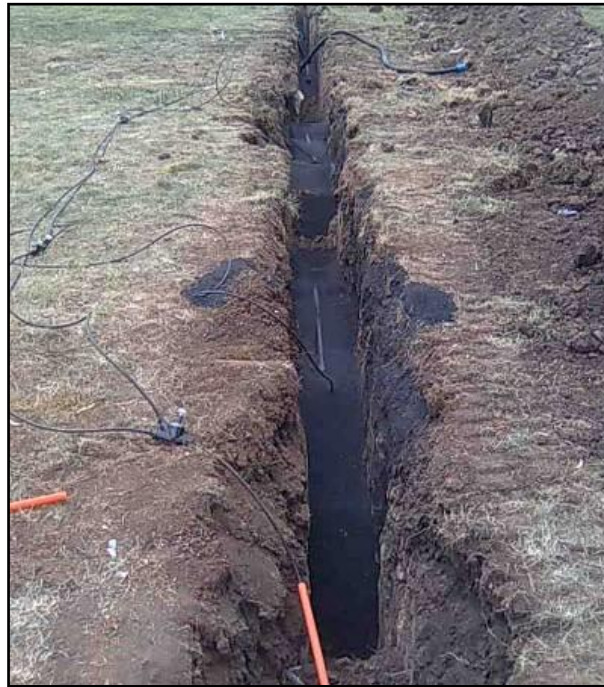
Figure 7: Large Anode Bed Installation (Multiple Anodes)
