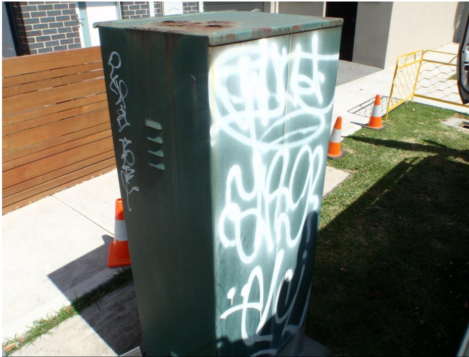
Figure 6: Deteriorated RTU Cabinet
