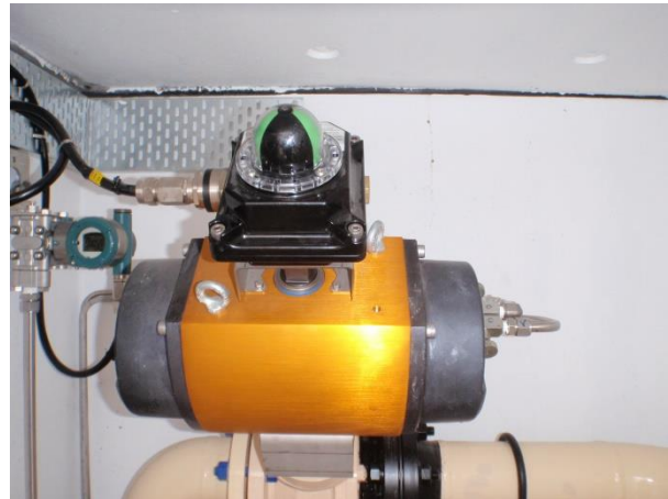
Figure 10: [C.I.C] actuator with rotary "dome type" switch type
