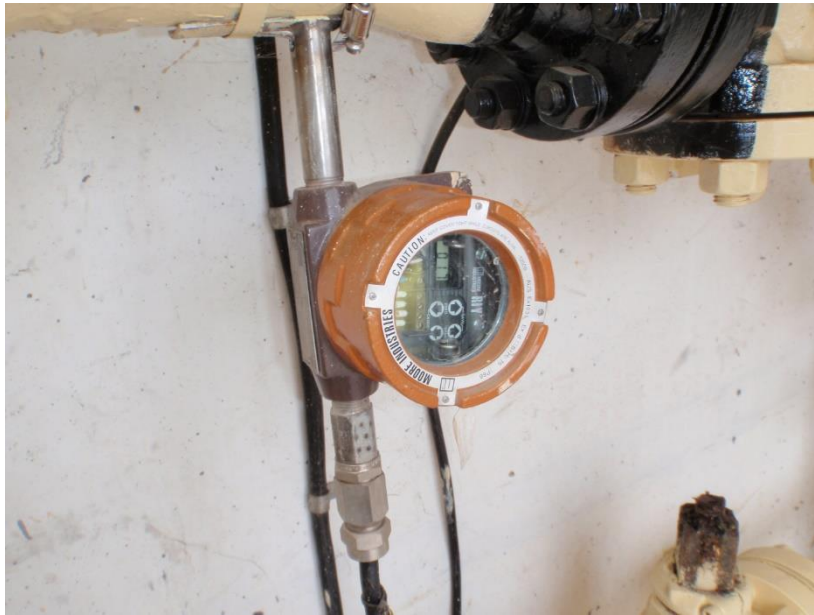
Figure 8: [C.I.C] Temperature Transmitter
