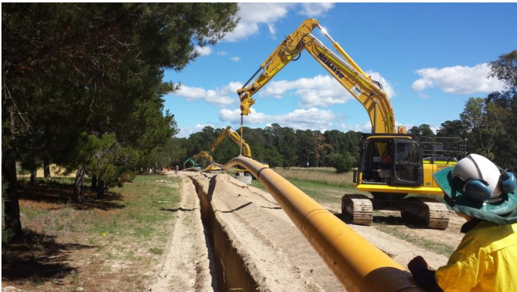
Figure 9–3: Secondary steel being laid for Hume Tuggeranong Interconnect (HTI) Stage 2.
