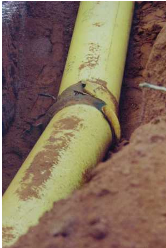
Figure 1. Buckling on the AGP caused by the TCK earthquake
