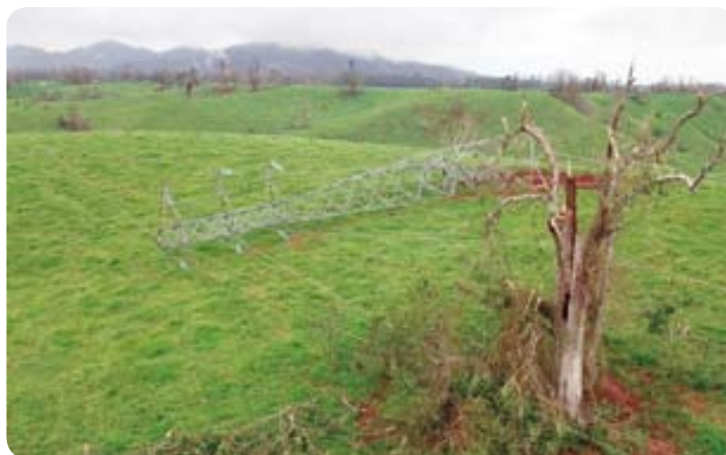
One of five transmission towers toppled by Cyclone Larry's destructive force.
