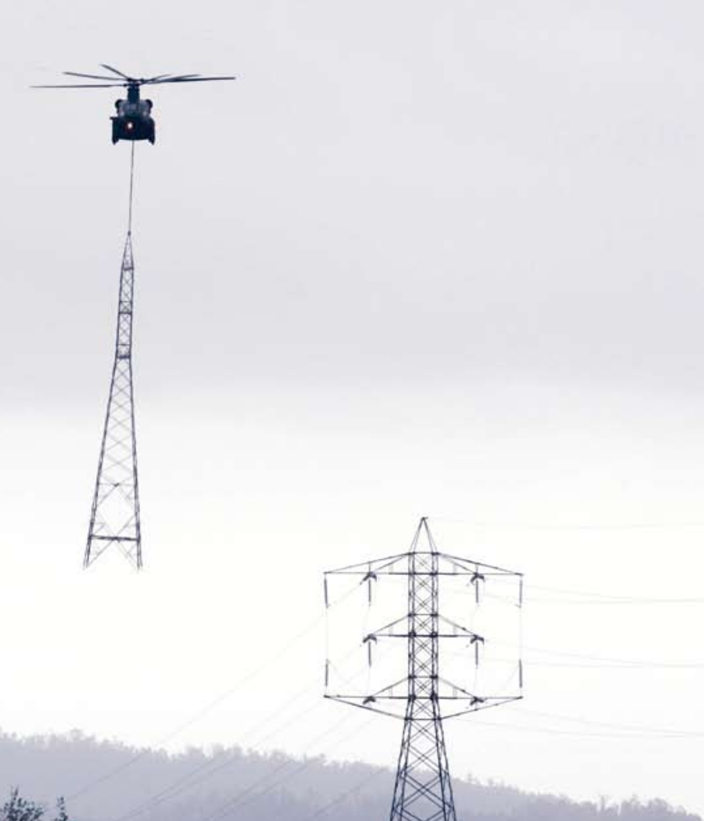
An Australian Defence Force Chinook helicopter air-lifts the transmission tower. Photograph courtesy of the Cairns Post.
