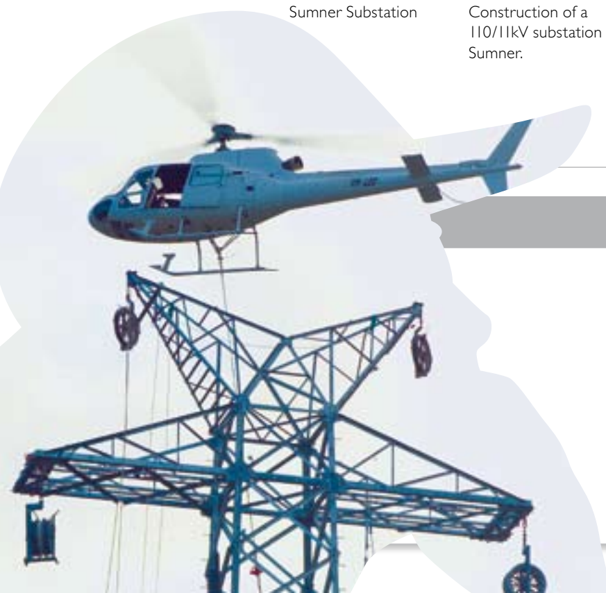
Helicopter stringing of the Belmont to Murarrie transmission line.
