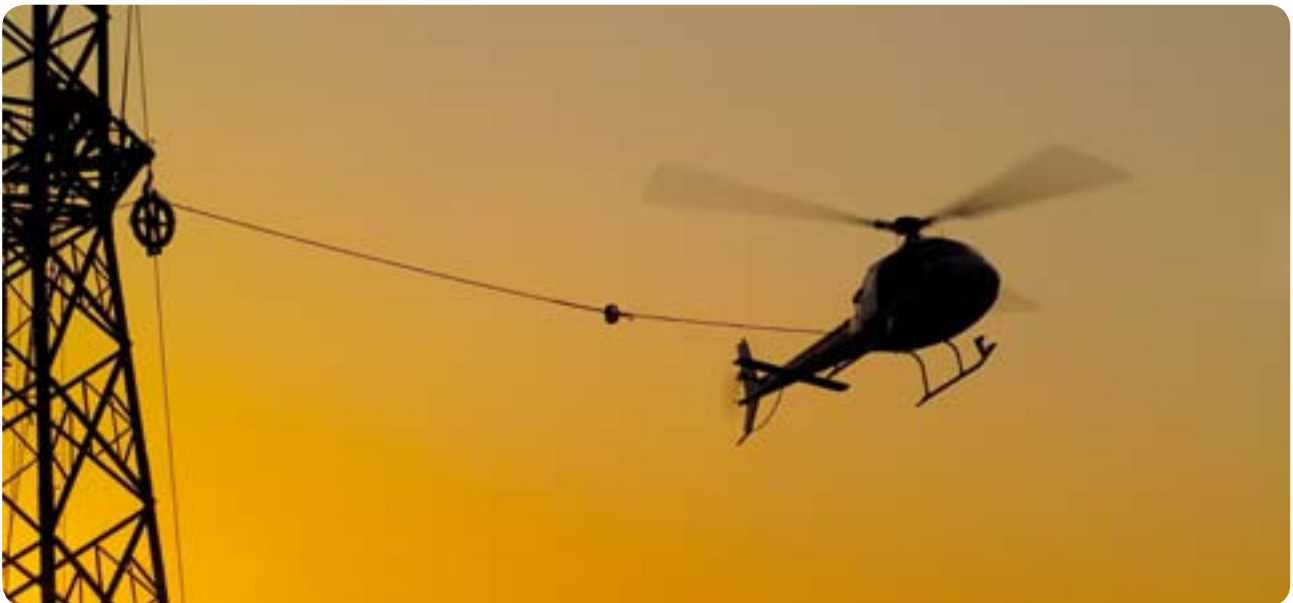
Helicopter stringing of the Belmont to Murarrie transmission line.
