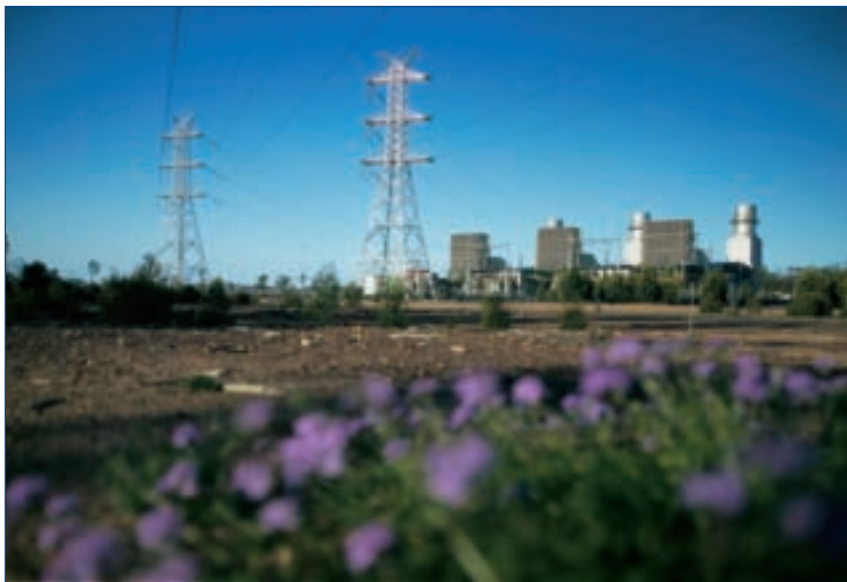
Powerlink's transmission line connection to Braemar Power Station near Dalby.
