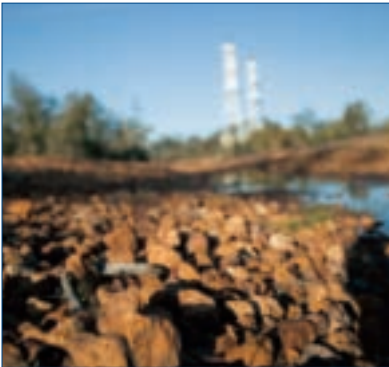
Powerlink's transmission line connection to Braemar Power Station near Dalby.
