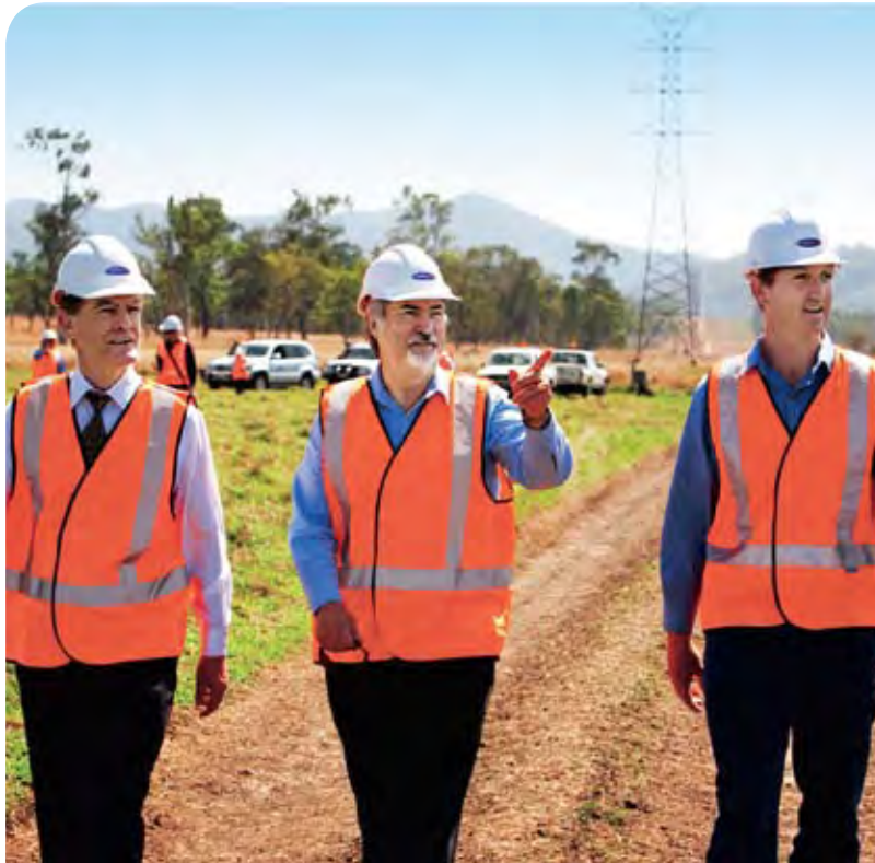
The Minister for Mines and Energy, Geoff Wilson MP (at left), with Gordon Jardine, Chief Executive and Eddie Van Der Draai, Construction Manager for the Nebo to Pioneer Valley transmission line project.
