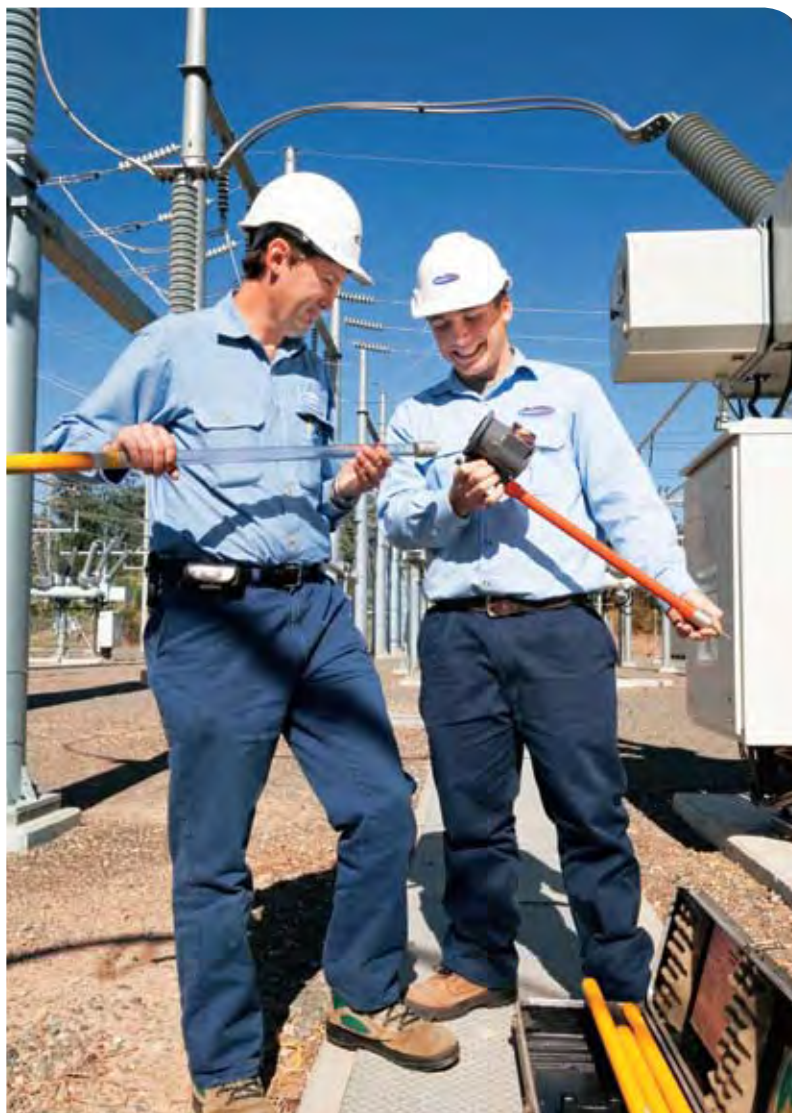
Above left: Warren Clayton, Systems Technologist, instructs Mark Quinlan, Electrical Apprentice, at Murarrie Substation, Brisbane.
