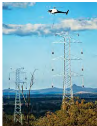
Helicopter stringing, used during construction of the Middle Ridge to Greenbank transmission line, helps to minimise environmental impact.
