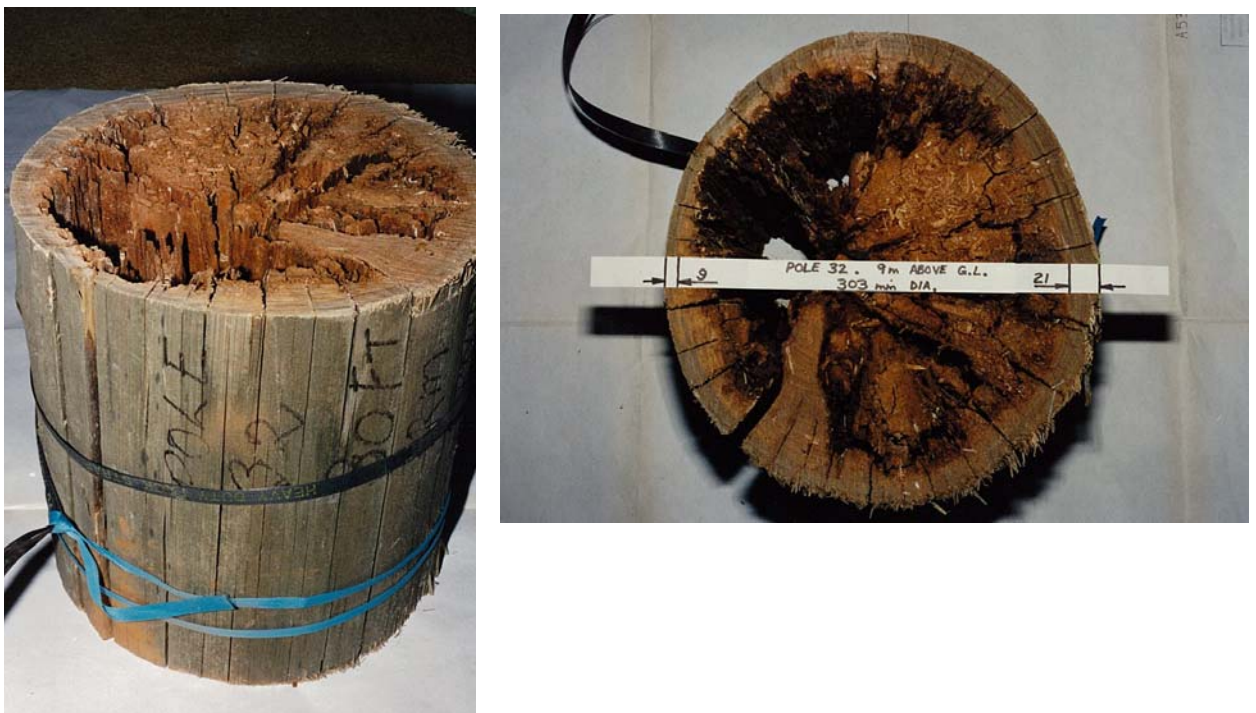
Figure 3 – Treated wood pole with fungal degradation 9 metres above ground line.
