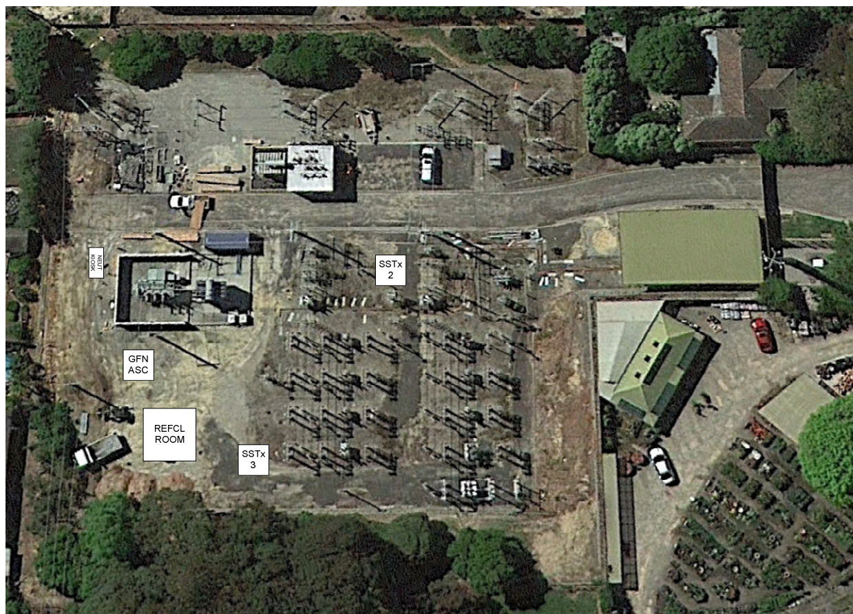
Figure 5: Aerial view of the RWN ZSS
