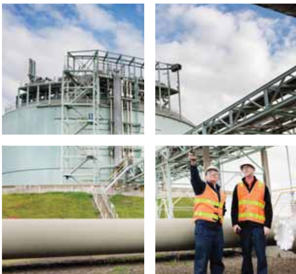
IMAGE: Dandenong LNG facility, Victoria, Tony Verde and Doug Dennis.
