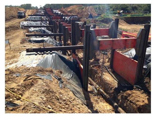
Temporary MOP restrictions were enforced on both pipelines while they were exposed during the project. The DN400 was lowered in service, with gas flowing in the pipeline. The DN250 pipeline required blow down, purging and cutting at both ends of the lowering section, due to pipe stress concerns in relation to the vintage girth welds, before lowering and tying-in the lowered pipe section to the existing pipe at either end with new tie-in spools.
