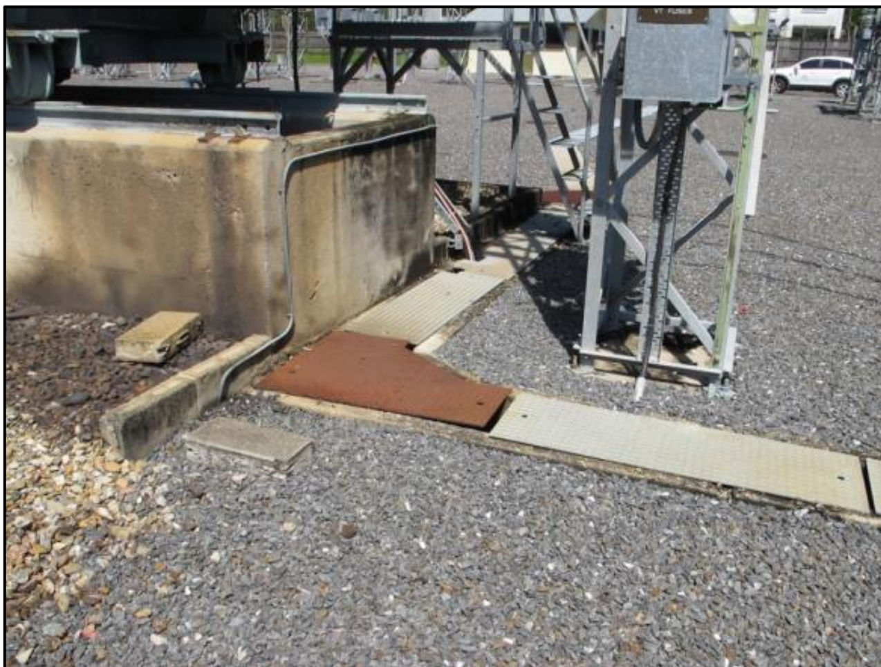
Figure 9 - Oil from leaking Transformer with no bund
