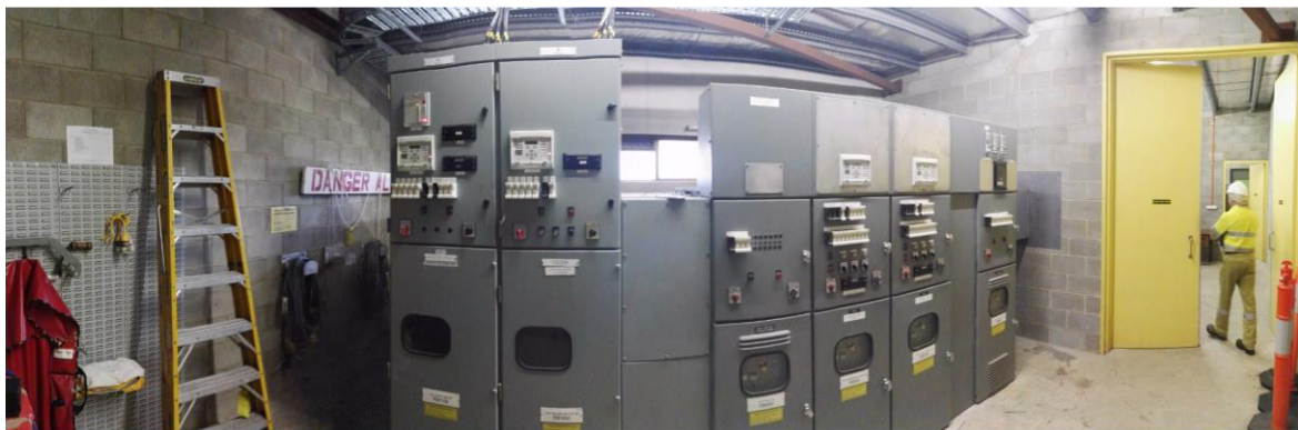
Figure A8 11 kV Switchboard Transformer 2 Bus
