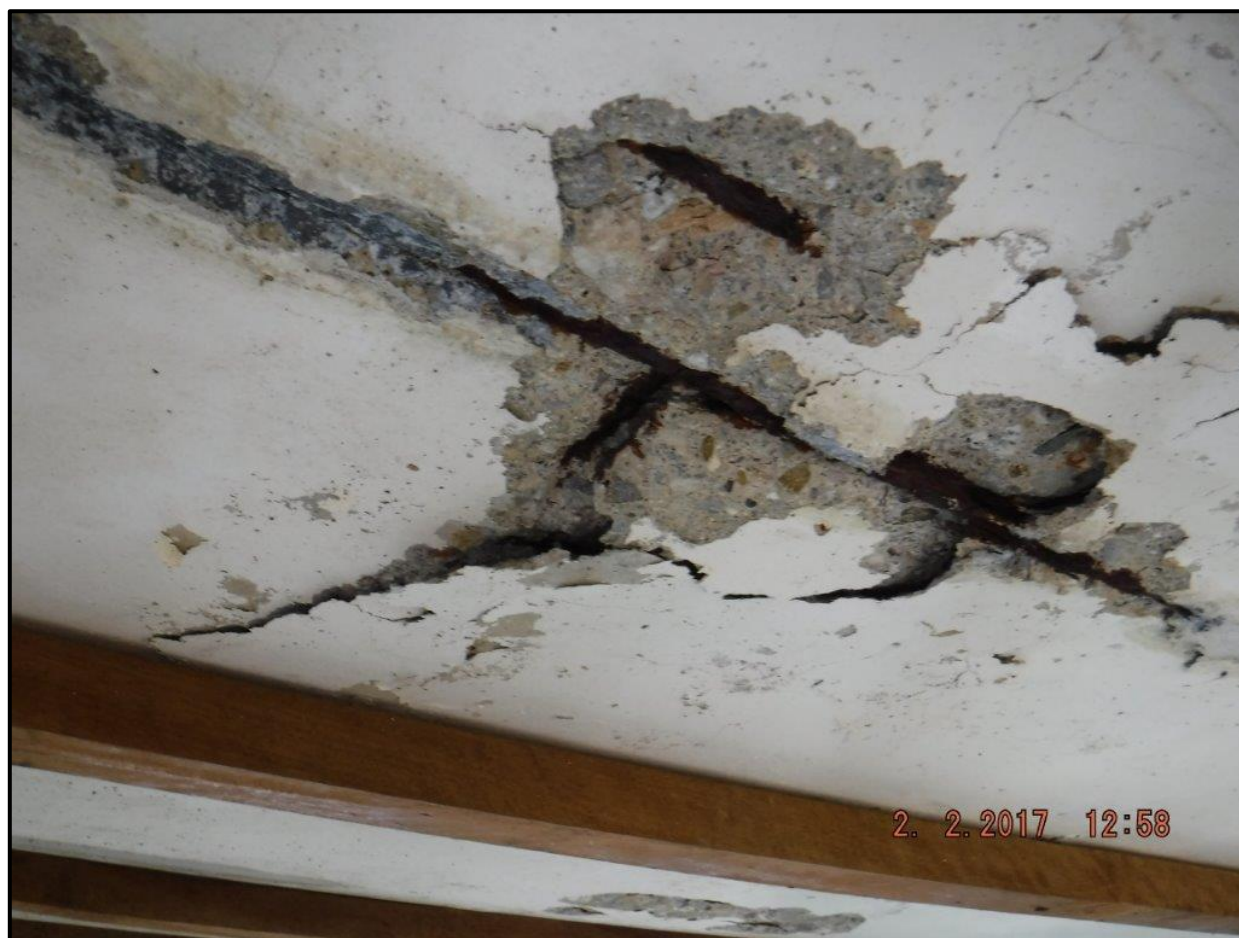
Figure 8- Spalling of concrete ceiling exposing fully corroded reinforcement
