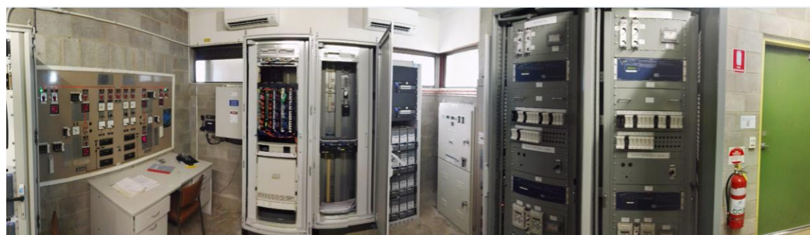
Figure A5 Control Room (No Spare Panel Space)
