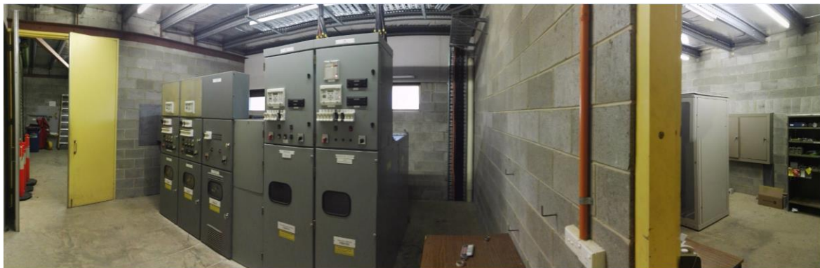
Figure A7 11 kV Switchboard Transformer 1 Bus
