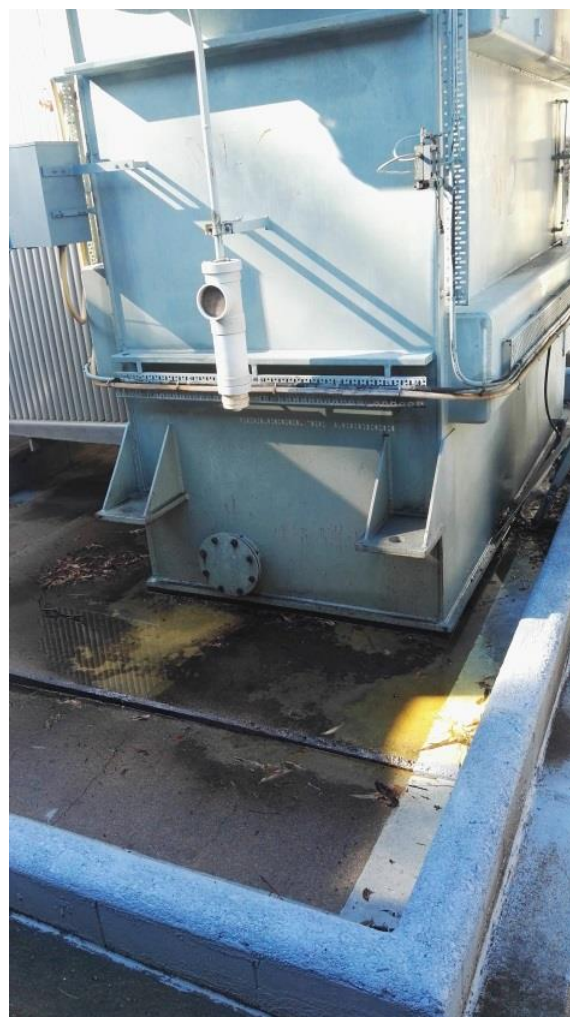
Figure A4 Transformer No. 2 Oil Leak
