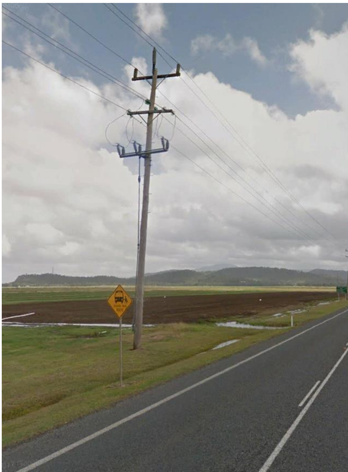
Figure A13 CANN-01 Typical O/H Build – Vertical Post Insulators
