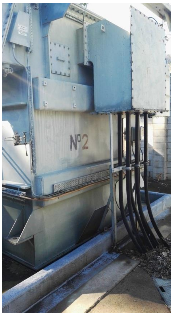
Figure A4 Transformer No. 2 Oil Leak
