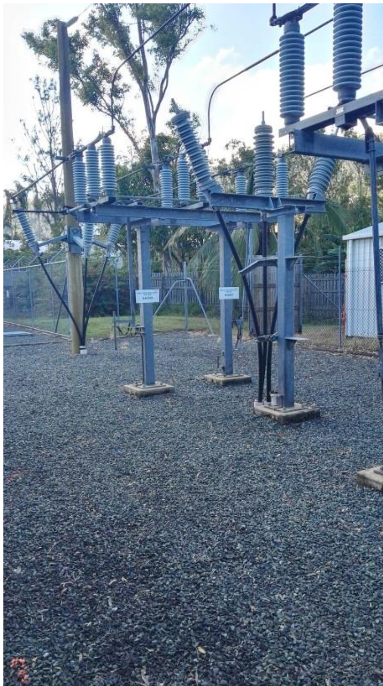
Figure A3 66 kV Feeder Tie (Failed CANN-01 Cable Out of Service – Droppers Removed)
