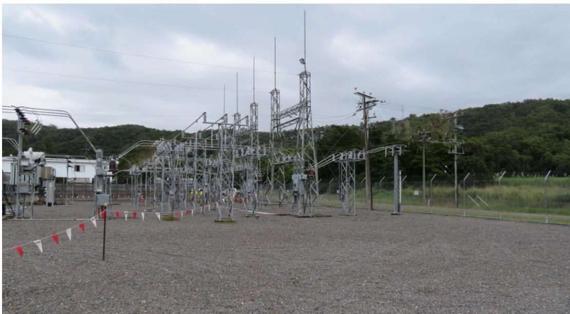
Figure 10 – 22 kV feeders and structures
