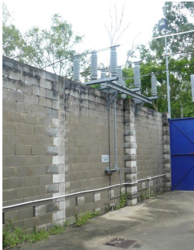
Figure A2: 66 kV Bus Tie Isolator ABS Operating Arm on the Other Side of Wall Adjacent that Cable Termination (Working Clearance Issues)
