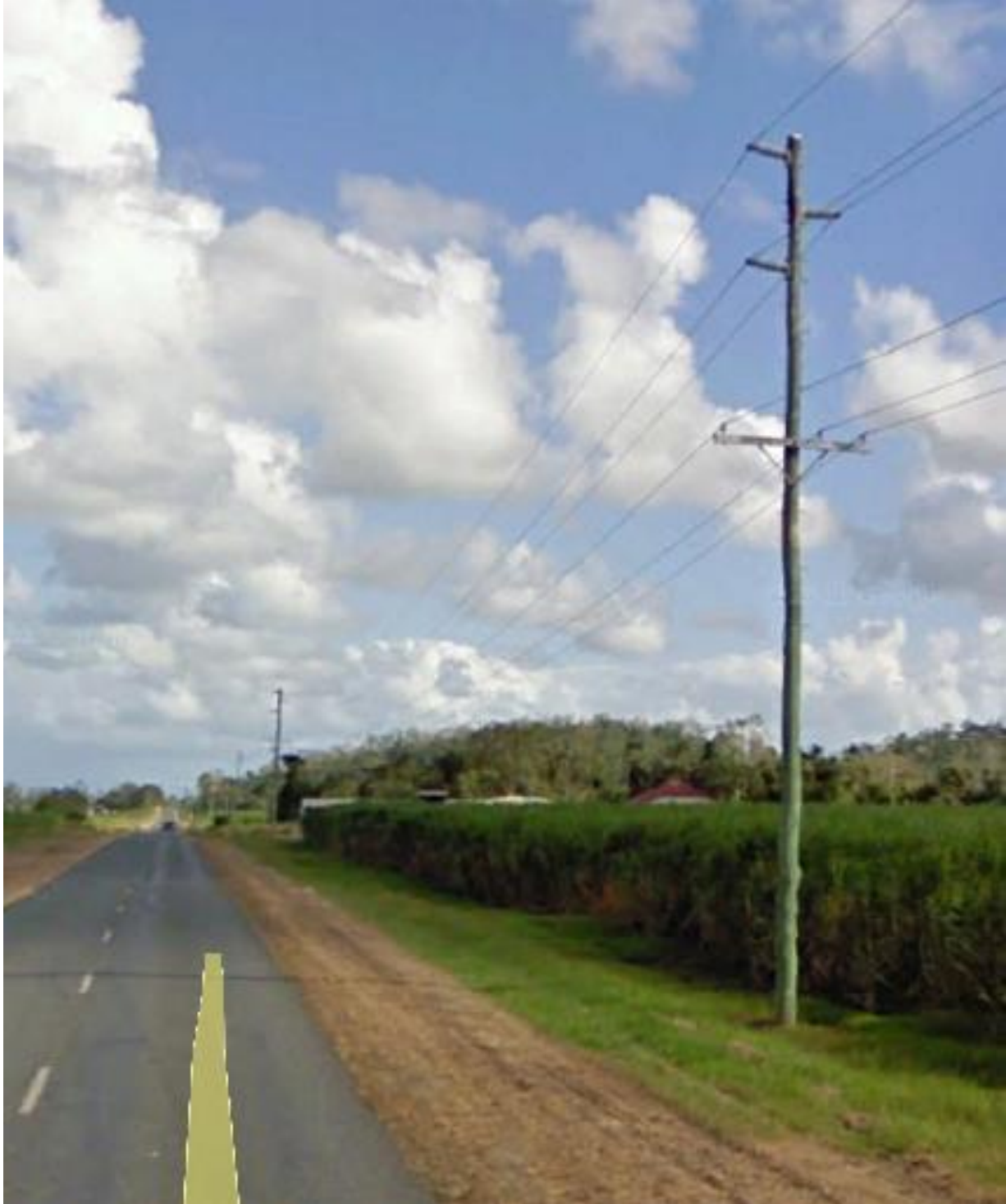
Figure A14 CANN-02 Typical O/H Build – Horizontal Post Stand-Off Insulators
