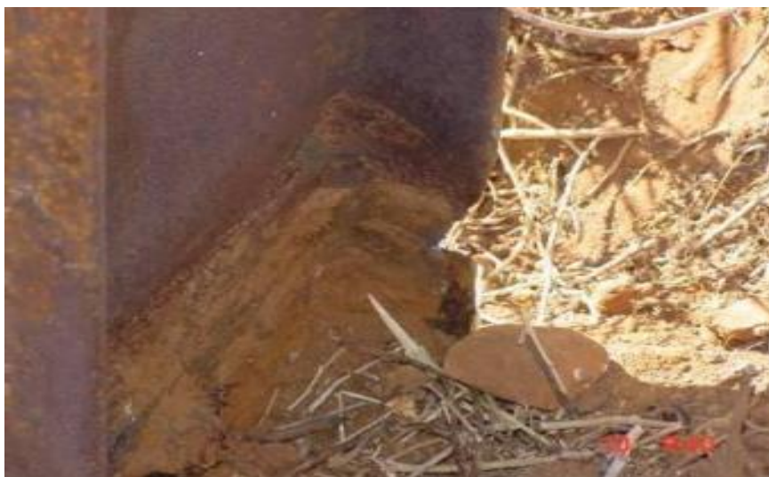
Image 6. Stobie Pole – Ground Line Corrosion
