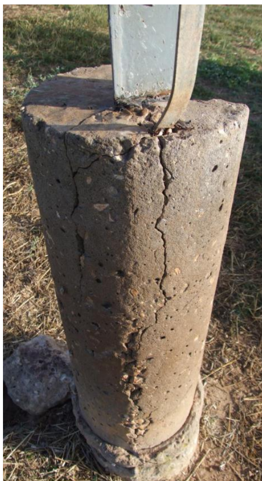
Image 7. Unreinforced and (Exposed) Foundation
