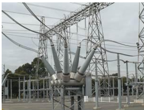
Figure 2 – 220 kV SF 6 CB
