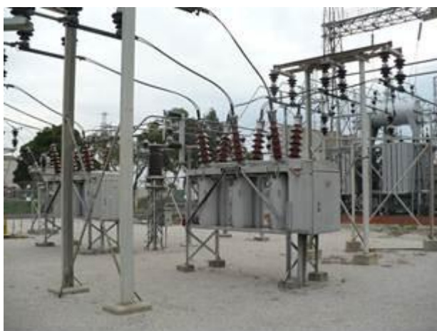
Figure 1 – 66 kV Bulk oil CB
