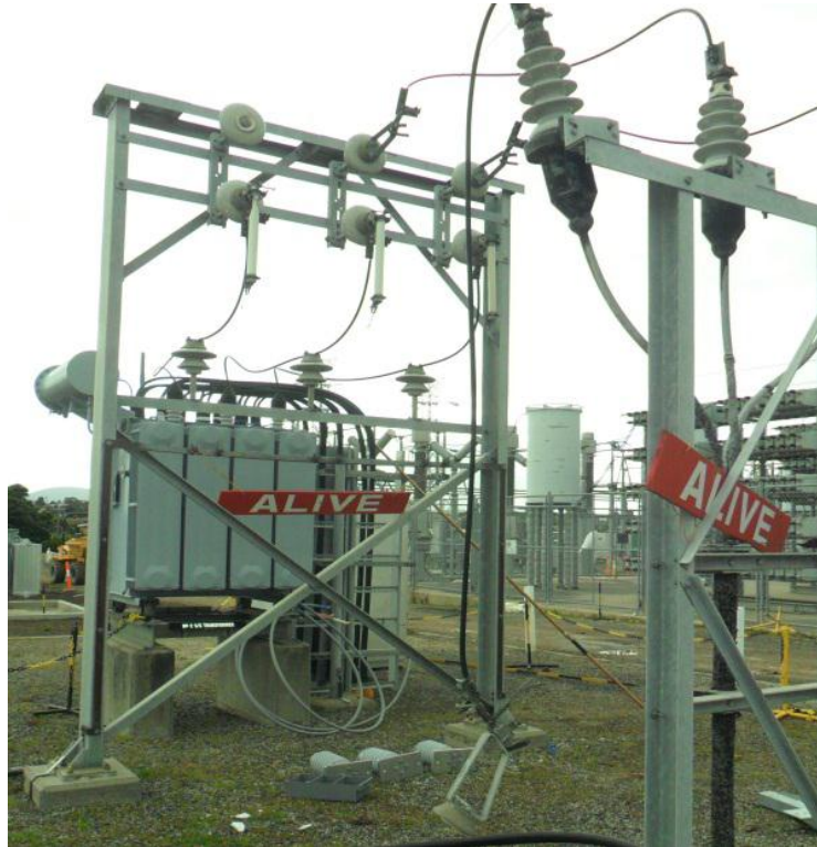
Figure 10 – ROTS 22 kV Station Service Transformer Fused Isolator Incident
