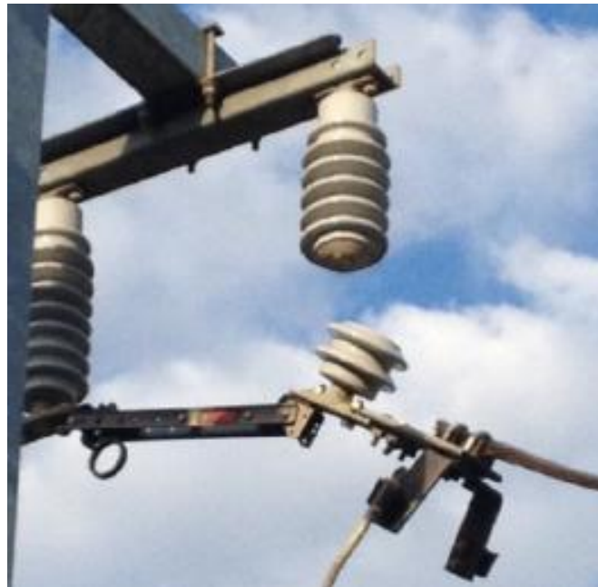
Figure 9 – Insulator Failure of an Underslung Disconnector
