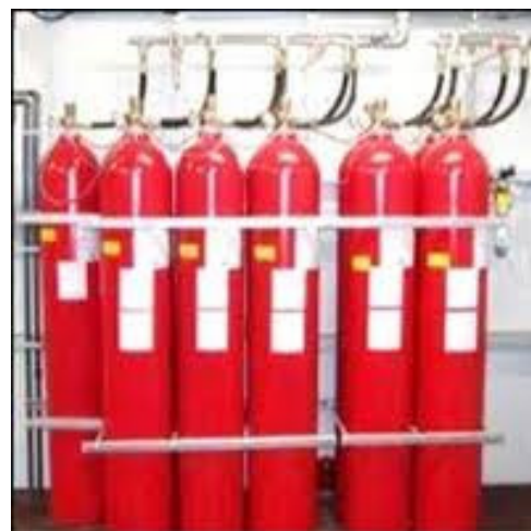
Figure 2 – Gaseous fire suppression system
