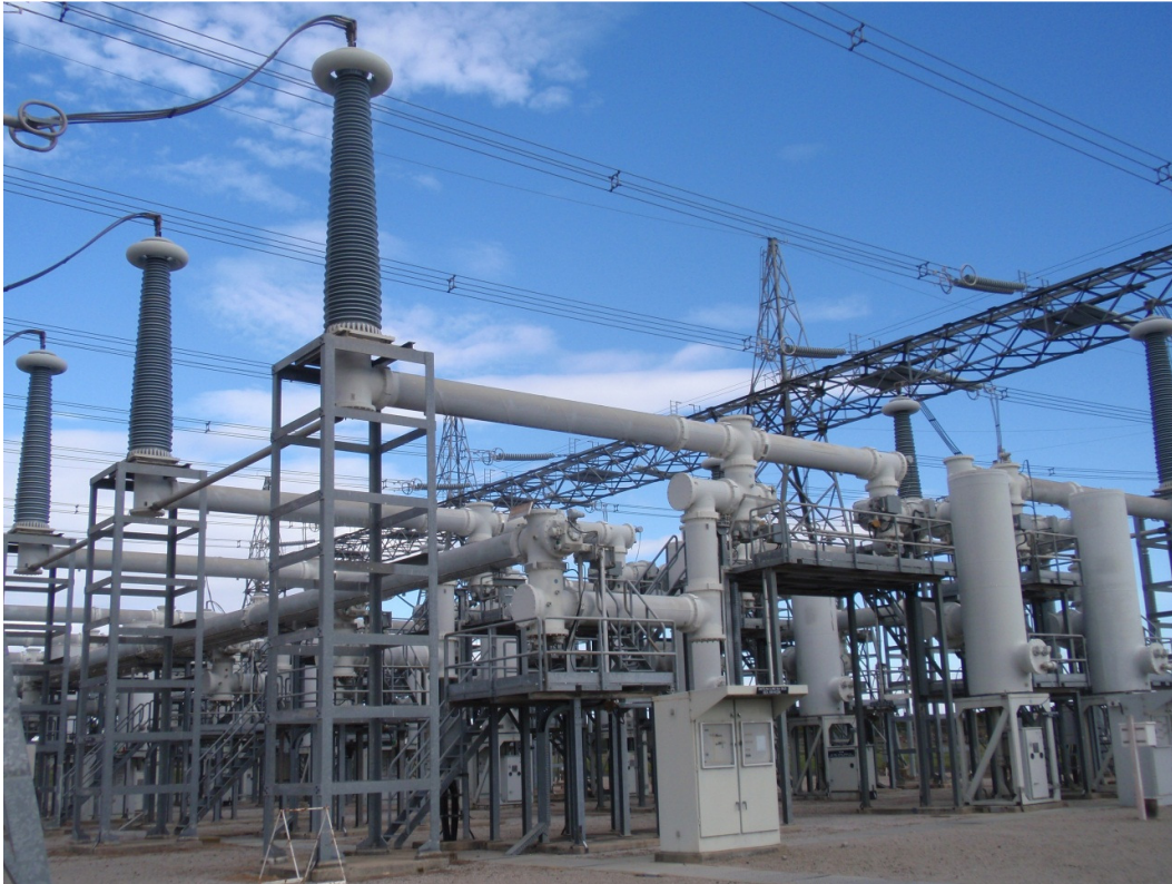
Figure 1 – GIS Equipment at SYTS
