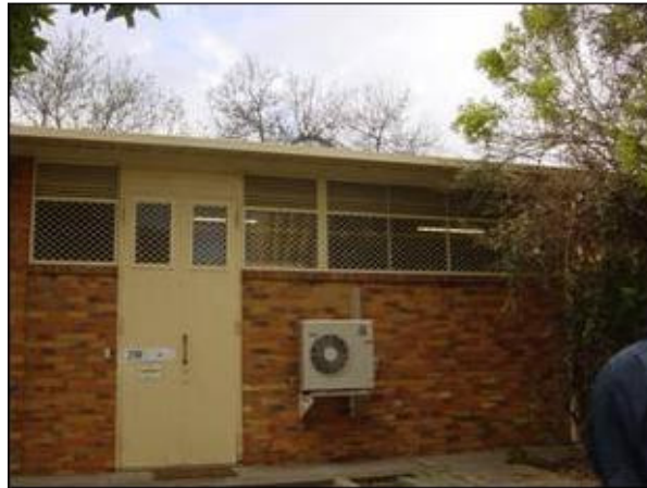
Figure 8 – [C.I.C] Existing Windows
