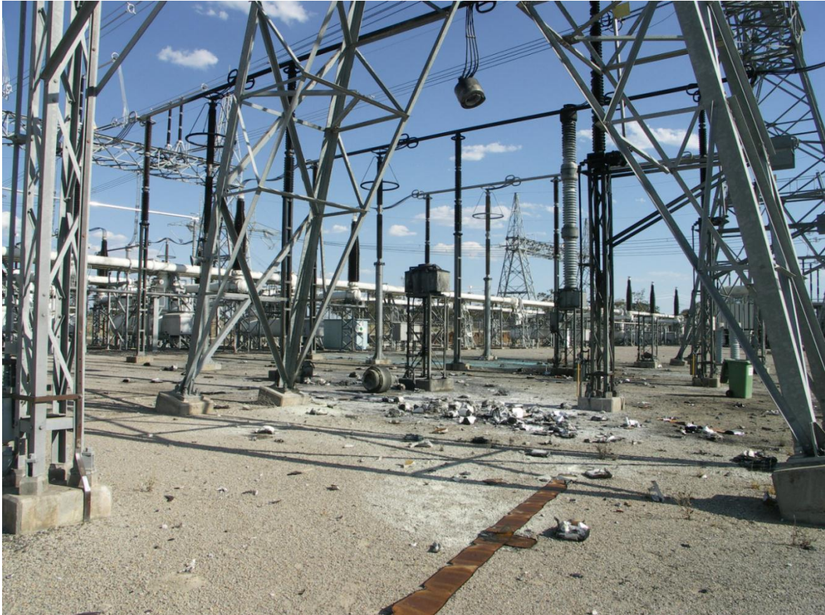
Figure 12 – 500 kV CVTCC Failure at SMTS (2009)
