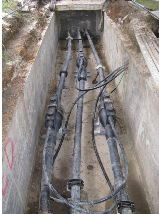
Figure 4 – Typical BTS-RTS Joint Bay (#12 shown) after cable joint replacement
