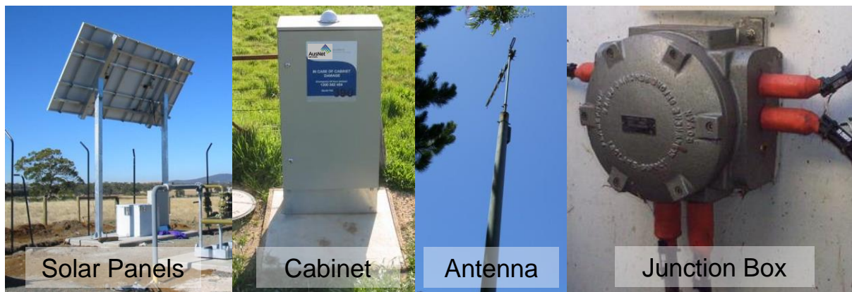
Figure 3: General SCADA Site equipment
