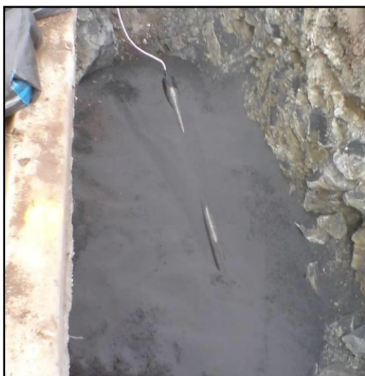
Figure 10: A Small Anode Bed Installation (Single Anode)
