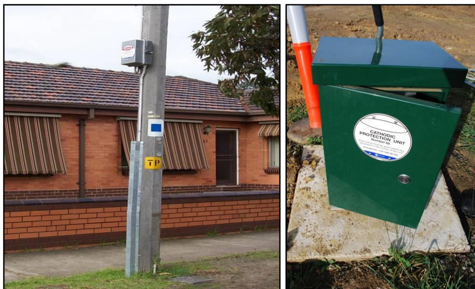
Figure 9: Typical CP Unit Installation
