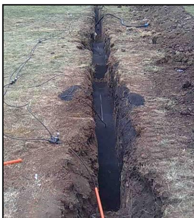
Figure 11: Large Anode Bed Installation (Multiple Anodes)
