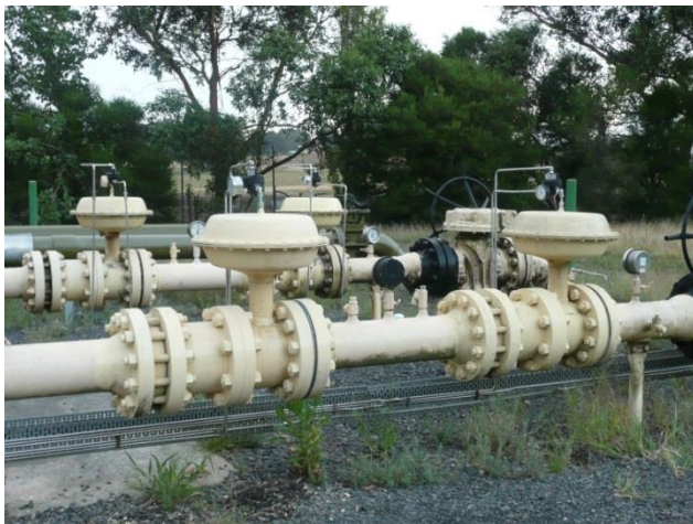
Figure 8: Ballarat CG Typical 2 leg wide open monitor configuration of Jet Stream Regulators
