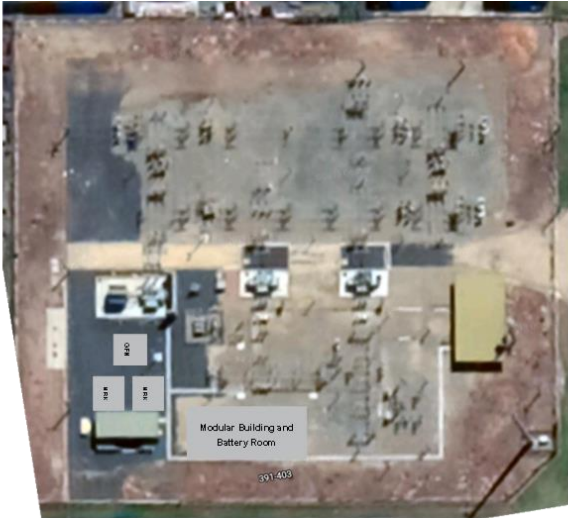
Figure 5: Aerial view of the SLE ZSS
