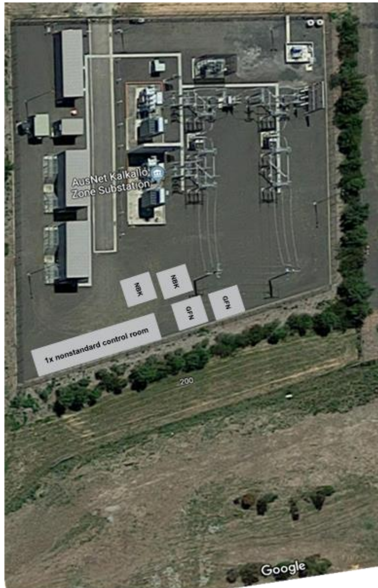
Figure 5: Aerial view of the KLO ZSS
