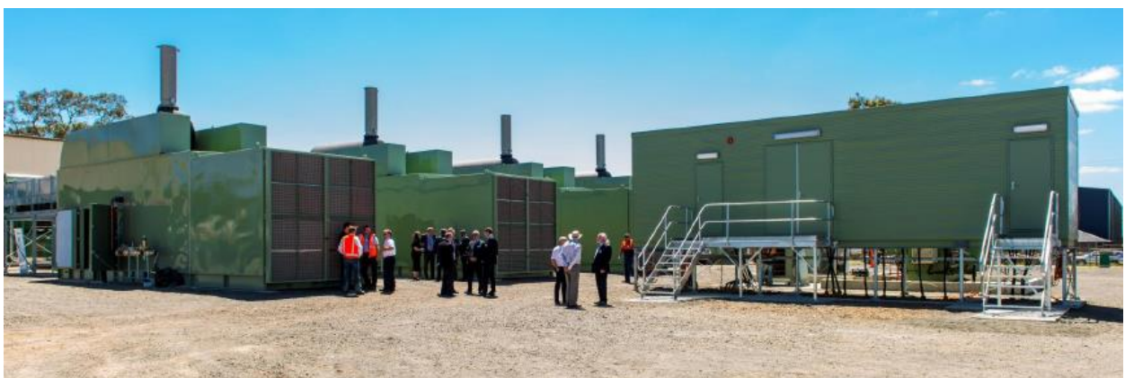
Figure 4 - Traralgon Power Station comprising 5 sets of 2 MW gas fired reciprocating engines
