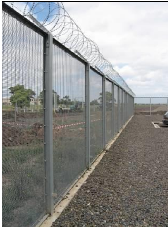
Figure 6 – Weldmesh Security Panel with Concrete Plinth and Barbed Tape
