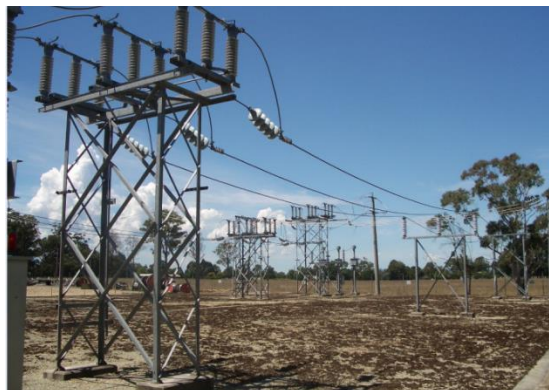
Figure 11 – Condition of switchyard surface at Numeralla zone substation (NLA)
