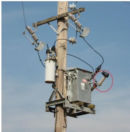
Figure 3 - Polymer housed surge arrester fitted to an isolating transformer
