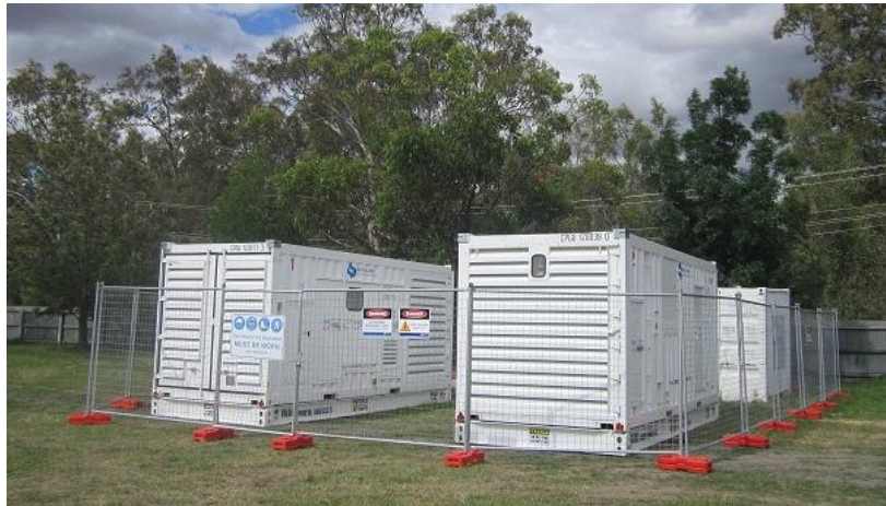
Figure 3 - Two sets of 1MW diesel generators and transformers supporting the BN1 feeder.
