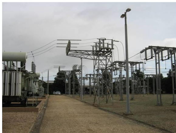
Figure 15 – Switchyard Lighting at Sale zone substation (SLE)
