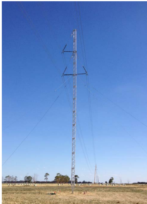
Figure 12 – An emergency restoration system stayed tower.
