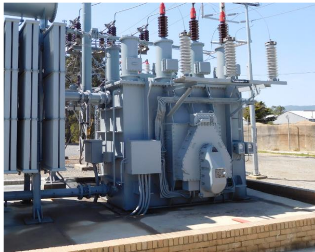
Figure 8 – Concreted bunded area at Bayswater zone substation (BWR)
