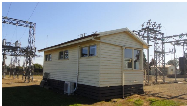
Figure 7 – Wood board clad control building at Warragul zone substation (WGL)
