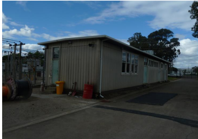
Figure 6 –Thomastown zone substation (TT) control building has ACM panels, transformer cubicles, etc.
