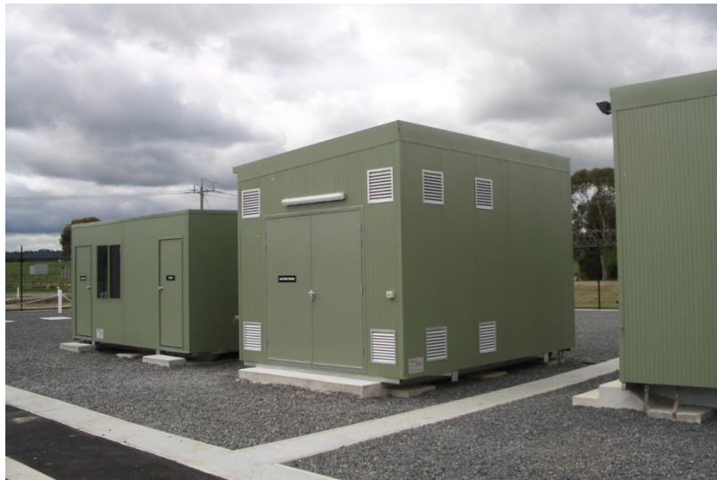
Figure 3 – Prefabricated buildings at Lysterfield zone substation (LYD)
