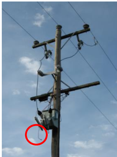
Figure 10 - Operation of an Earth Leakage Disconnect
