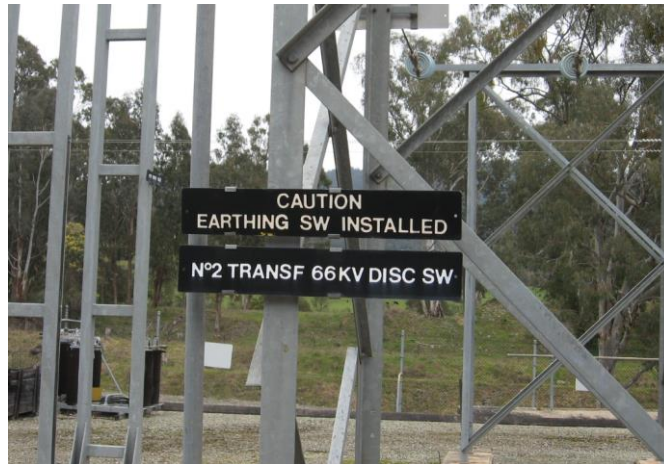
Figure 17 – Operational nameplates at Mount Beauty zone substation (MBY)
