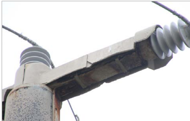
Figure 9: Steel Crossarm rusting under an animal cover
