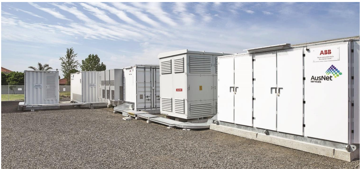
Figure 6 - Example layout of a grid-scale battery storage system with generator backup (image courtesy of ABB Australia)
