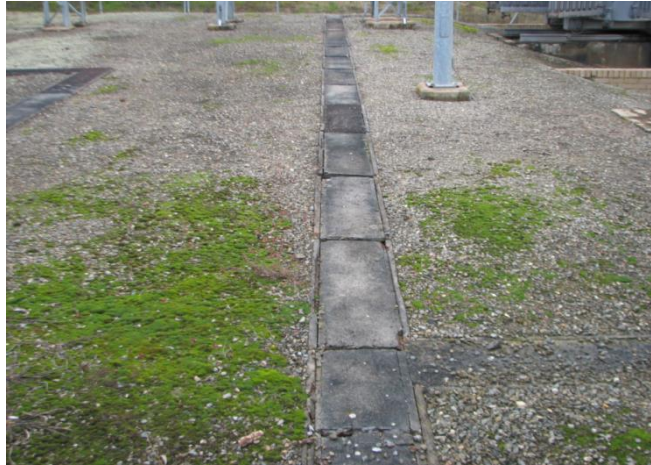
Figure 16 – Cable trench and cover lids at Mount Beauty zone substation (MBY)
