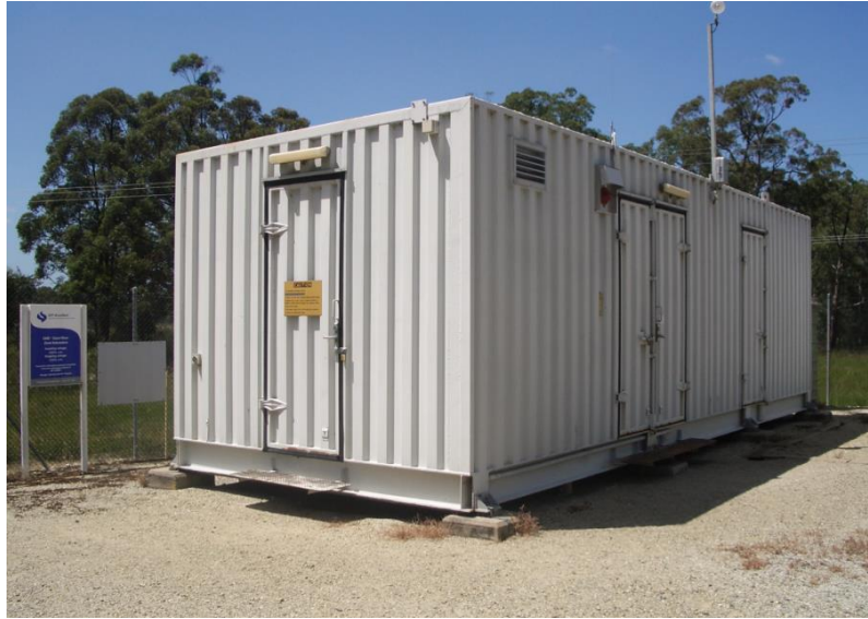
Figure 4 – Shipping container type control building at Cann River zone substation (CNR)
