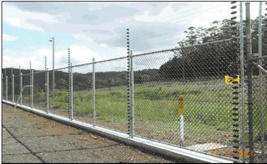
Figure 7 – Electric Power Fence inside Chain Wire Mesh Fence
