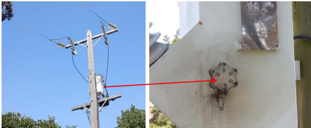
Figure 11: Distribution Transformer Tap Setting
