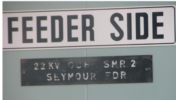
Figure 19 – Faded nameplates at 22 kV Switchyard Seymour zone substation (SMR)
