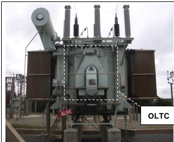
Figure 1 – Typical Zone Substation Power Transformer with OLTC
