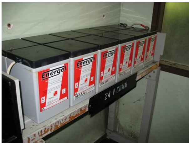
Figure 3 – Flooded Lead Acid Battery
