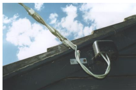
Figure 3 – Grey PVC Service & 'Dog-bone' Termination Fitting
