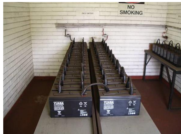
Figure 4 – Valve Regulated Lead Acid Gel Battery
