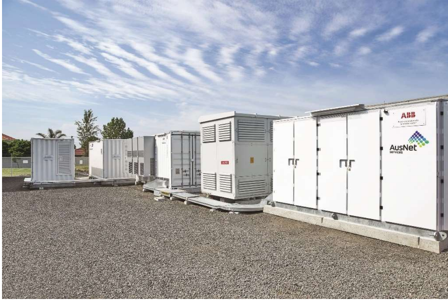
Figure 4 The GESS, installed and operational. Battery containers are in the background, with the inverter, transformer and switchgear containers in the foreground.
