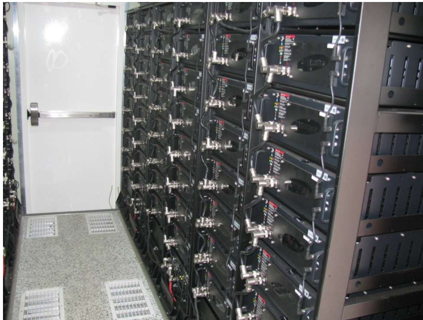
Figure 5 Battery container view from inside.
