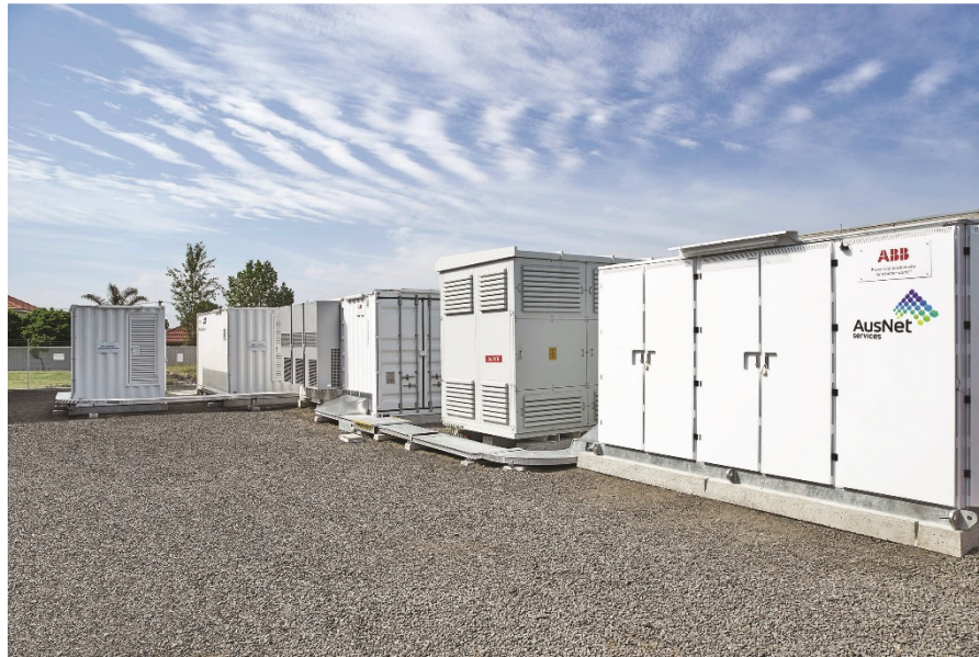
Figure 3 The GESS, installed and operational. Battery containers are in the background, with the inverter, transformer and switchgear containers in the foreground.
