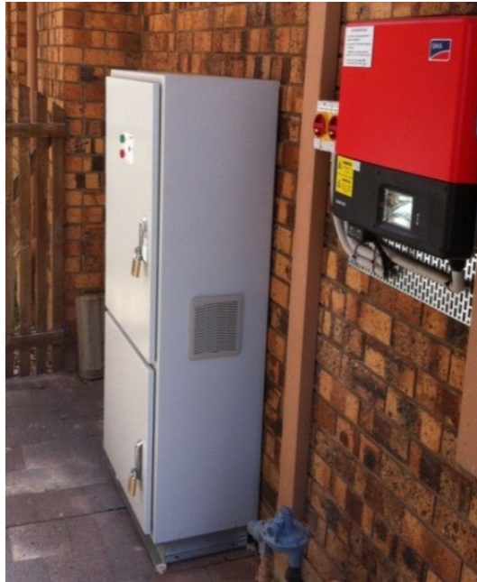
Figure 4.1 An installed Residential Battery Storage System (batteries in lower compartment of cabinet, inverter/charger and control system in upper compartment), and wall-mounted solar inverter.
