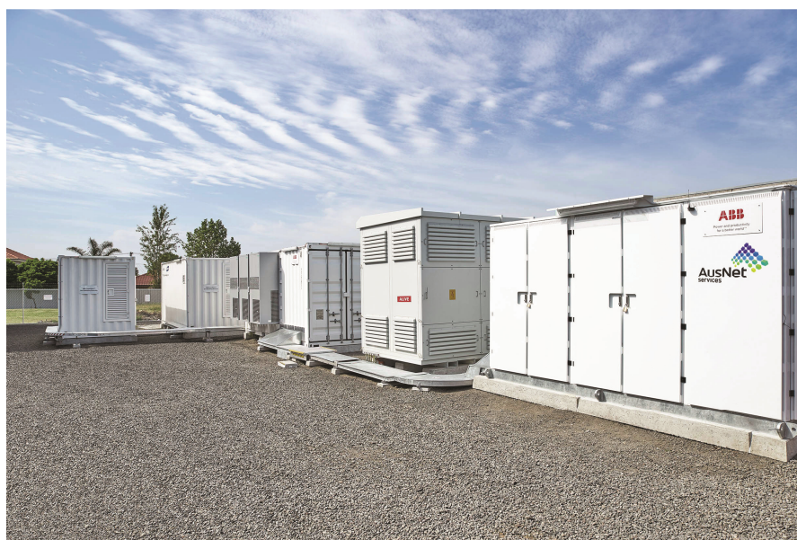
Figure 5.1 The GESS, installed and operational. Battery containers are in the background, with the inverter, transformer and switchgear containers in the foreground.
