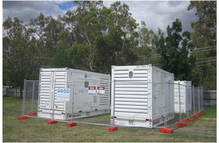
Above. Two sets of 1MW diesel generators and transformers supporting our network in Euroa.
