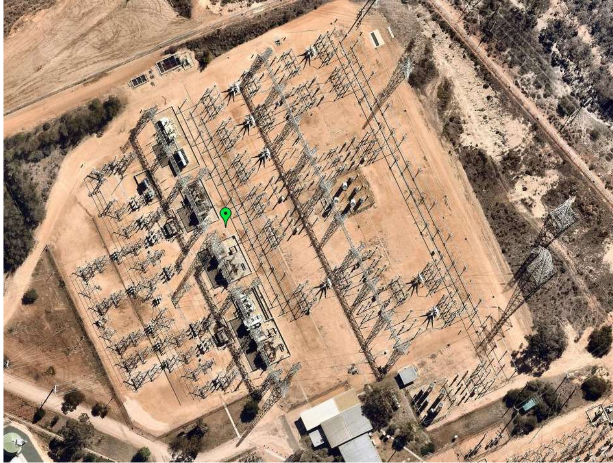
Figure 2 – Red Cliffs Terminal Station Aerial View
