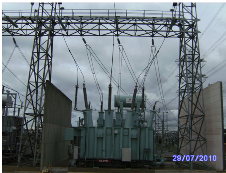
Figure 4 – Gantry legs within bunded areas at RWTS
