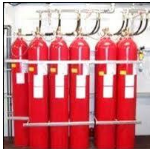
Figure 2: Gaseous fire suppression system
