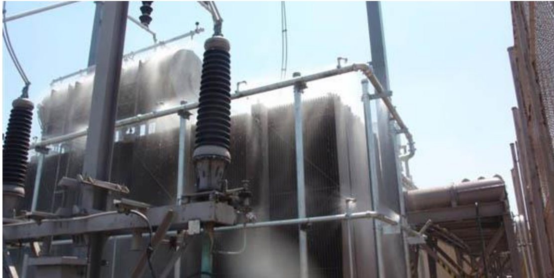
Figure 3 – Water deluge system operating on a power transformer
