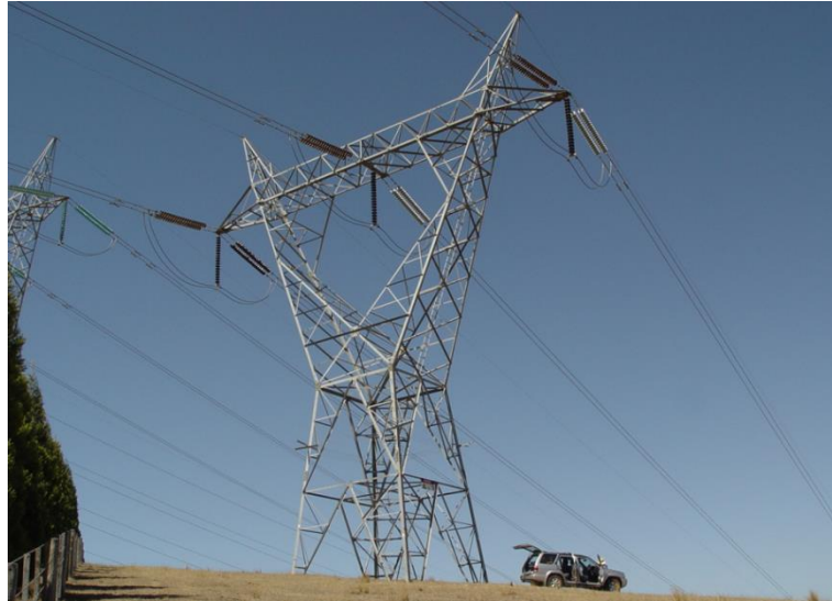
Figure 5 - DDTS-SMTS No. 1 330 kV strain tower
