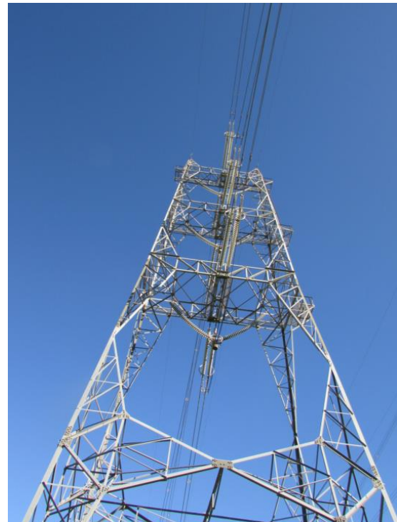
Figure 7 - HWTS-CBTS No. 4 500 kV transposition tower
