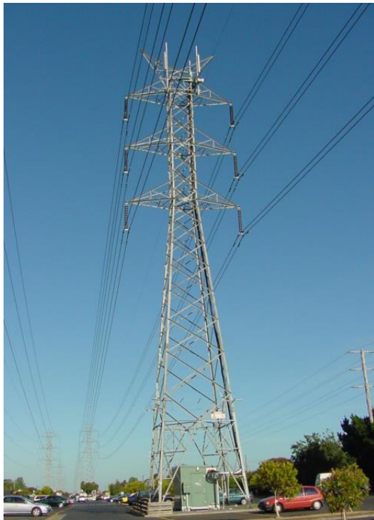
Figure 6 - ROTS-SVTS 220 kV suspension tower
