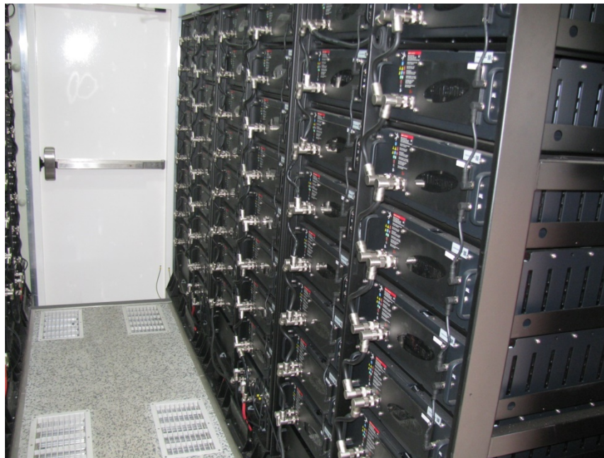
Figure 5.2 Battery container view from inside.
