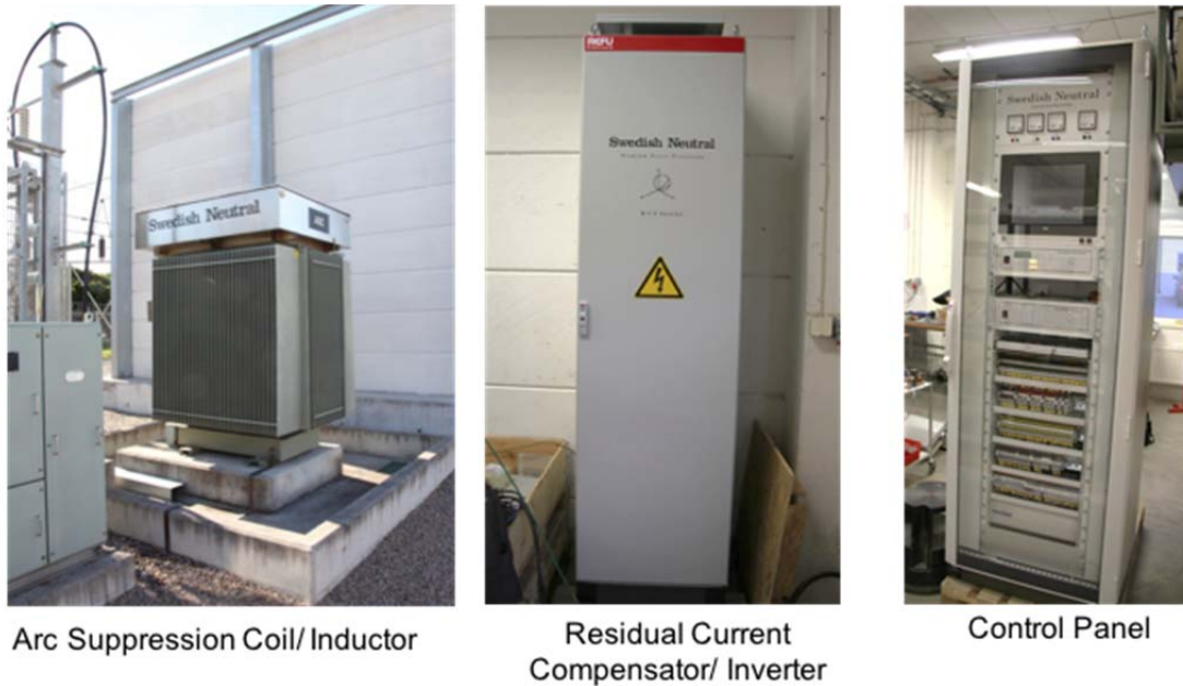
Figure 3: Three components to REFCL technology
